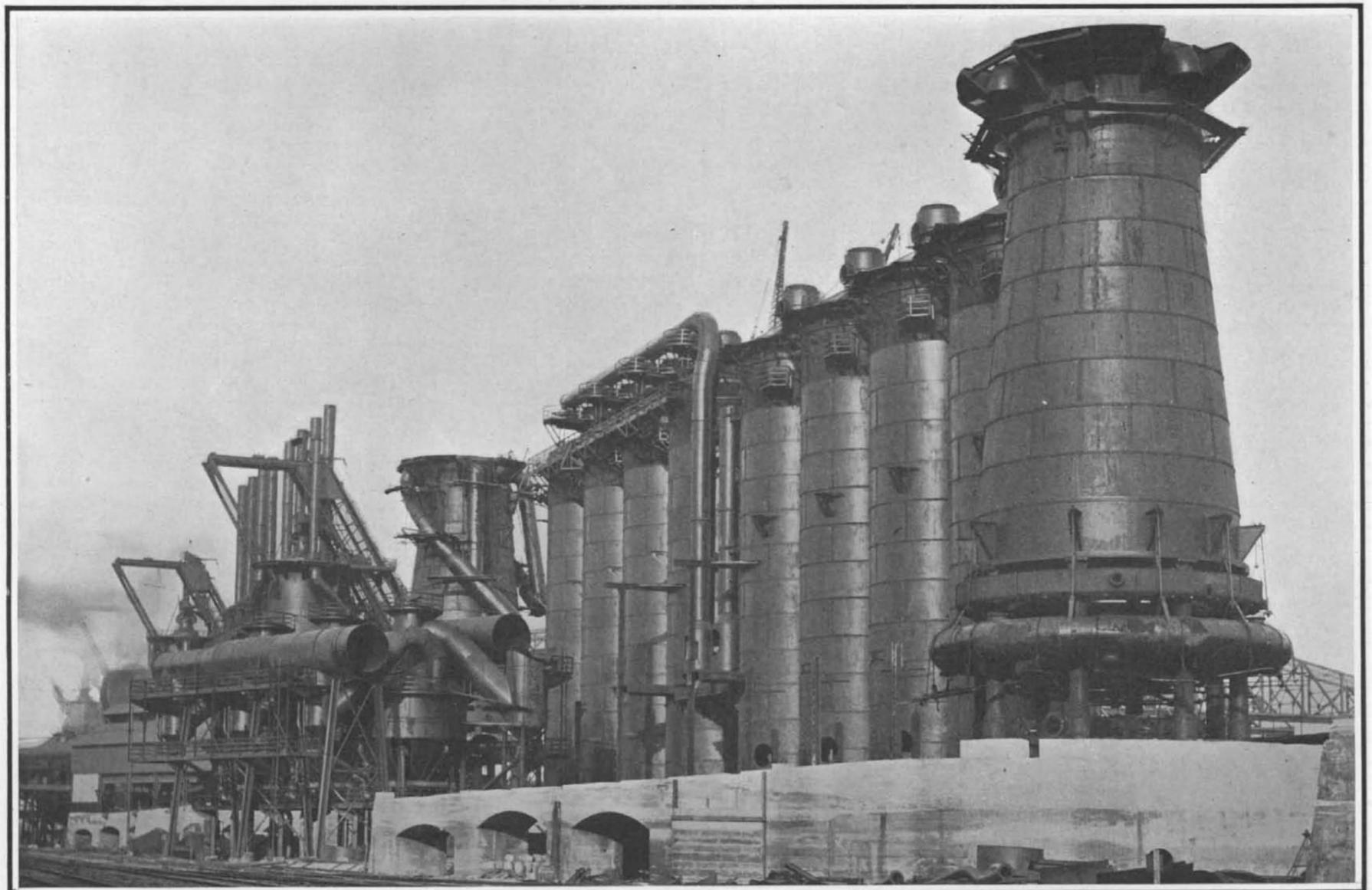
The 450-ton furnaces, hot stoves, and gas-cleaning plant in course of erection. The completed works will include 16 of these furnaces and accessories, capable of producing annually 2,400,000 tons of pig iron.
