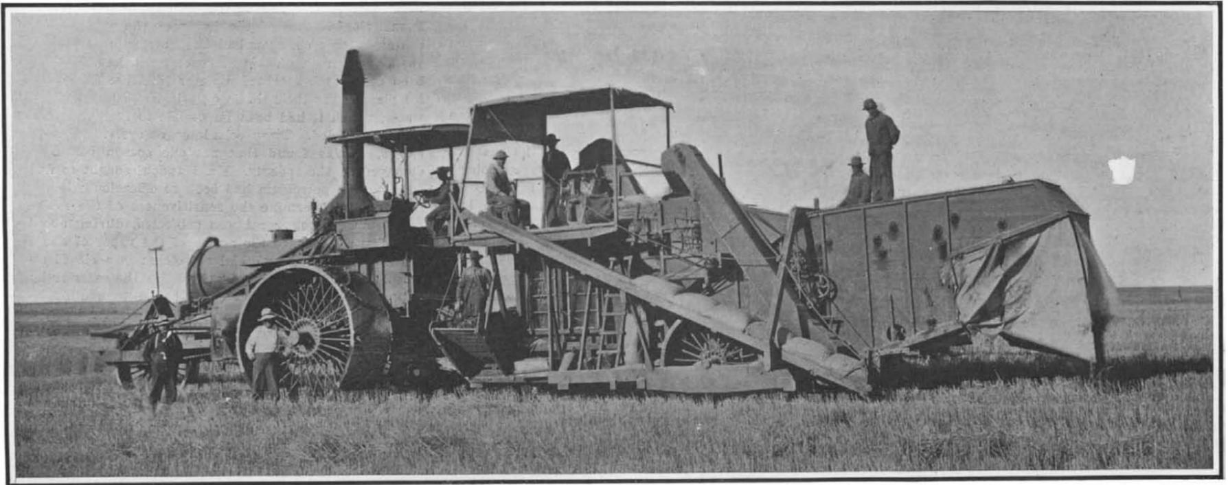
This machine cuts the wheat, threshes it, and delivers it ready sacked in one continuous operation.
