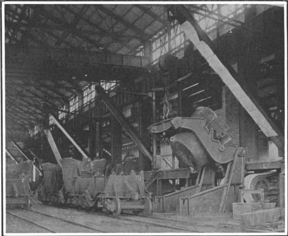
The molten iron from the furnaces is brought to the open hearth furnaces in 60-ton ladles, one of which
