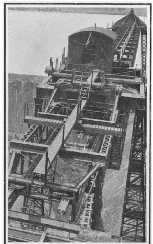
Shows details of Brown hoisting machinery. Length, 354 ft. 8 in.; bucket lifts 7½ tons.
