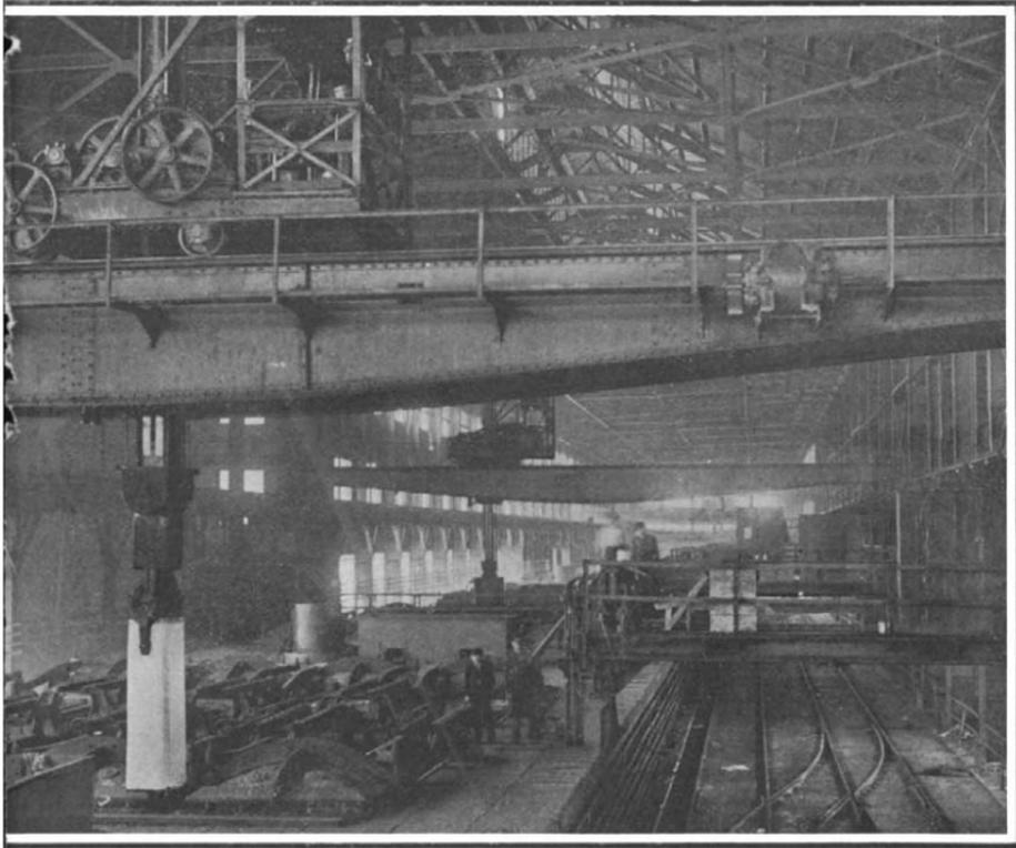
Here the ingots are heated in gas-fired underground furnaces to the proper temperature for rolling.
