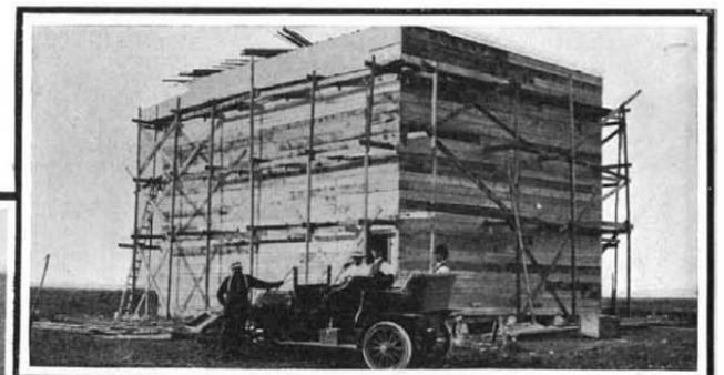
TYPE OF ELEVATOR ERECTED ON IDAHO RANCH FOR INDIVIDUAL USE. FROM THESE ELEVATORS THE GRAIN IS SHIPPED BY RAIL.
