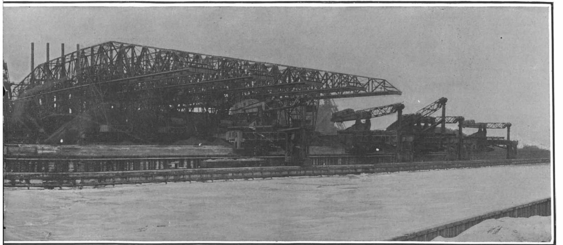
Five traveling conveyer bridges for transporting the ore to stock yard and furnaces.
