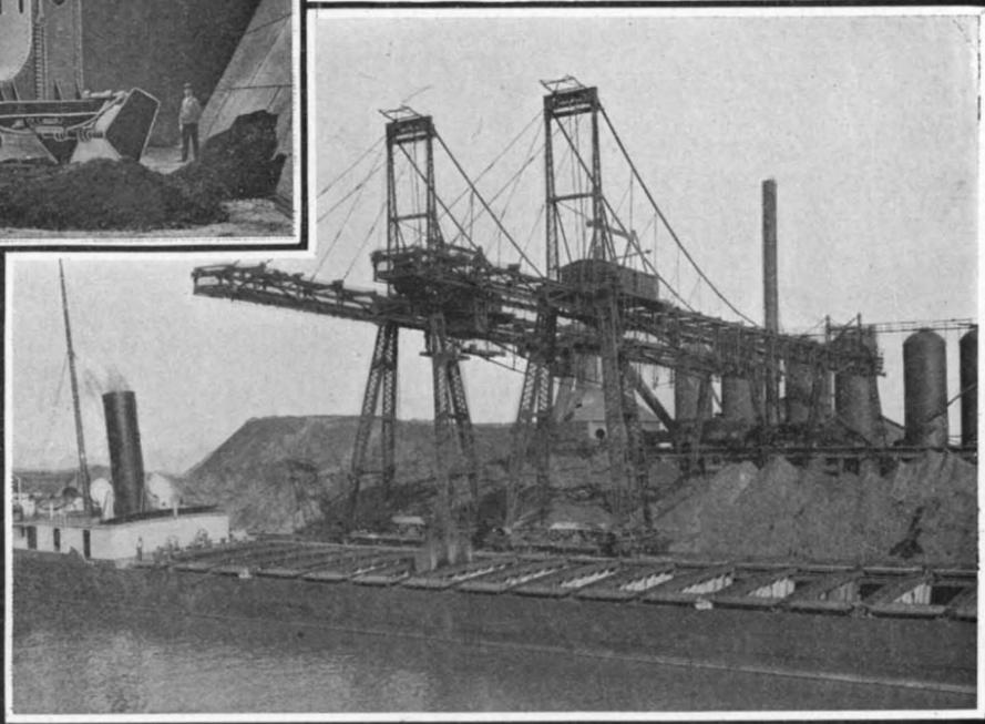
Length of tramway, 360 feet. Bucket capacity, 5 tons.
