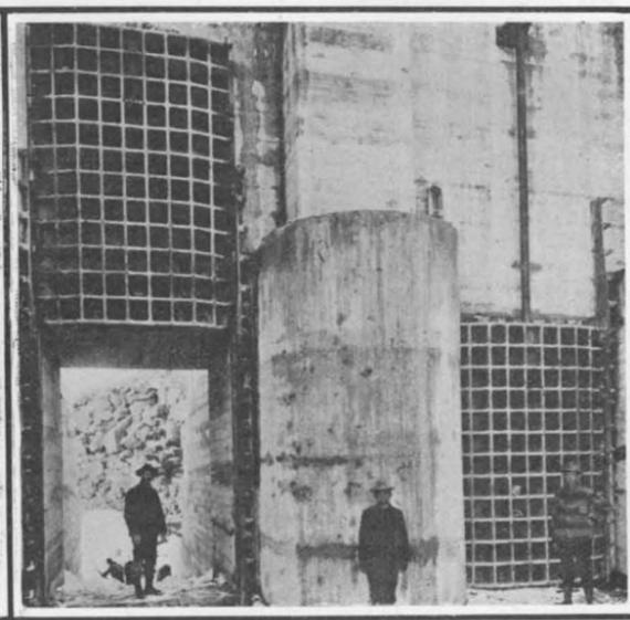
This view shows 22,000 second-feet passing through five 8 x 12 foot gates and five large and two small penstock openings in diversion channel. Two of the 8 x 12-foot coffin gates in diversion channel dam. MINIDOKA PROJECT, IDAHO.
