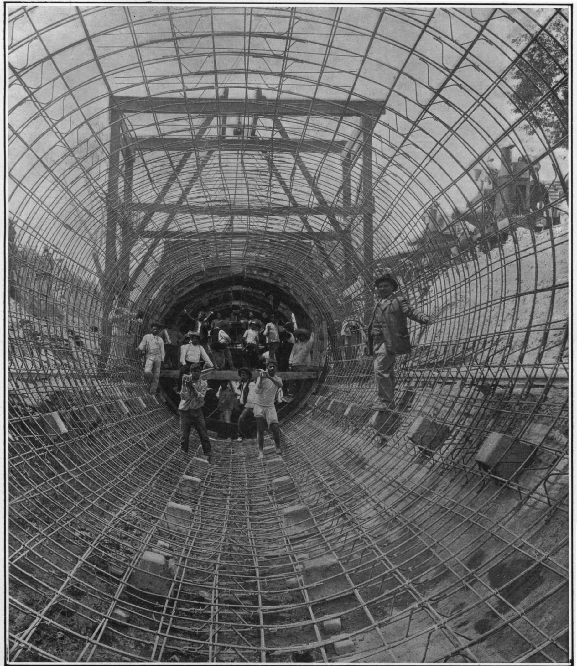
LOOKING THROUGH A REINFORCED CONCRETE CONDUIT IN COURSE OF CONSTRUCTION.—[See page 328.]
