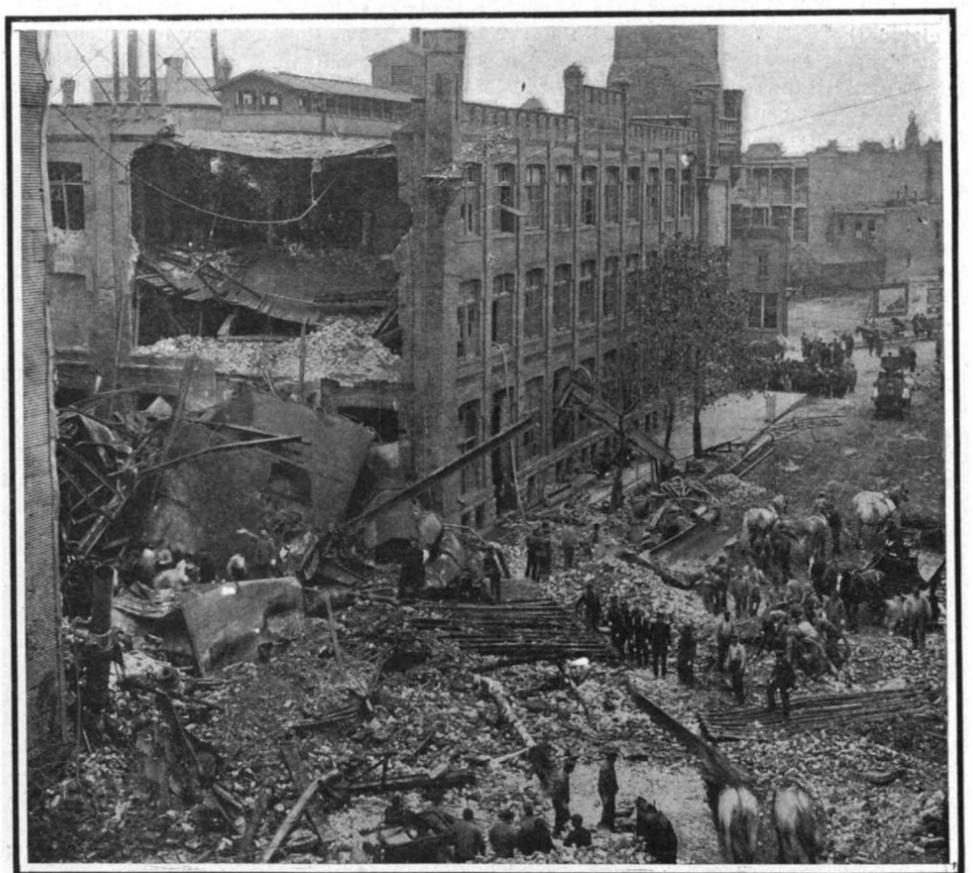
To the left is seen the wall of the building 60 feet high which was moved bodily a distance of 4 feet.
