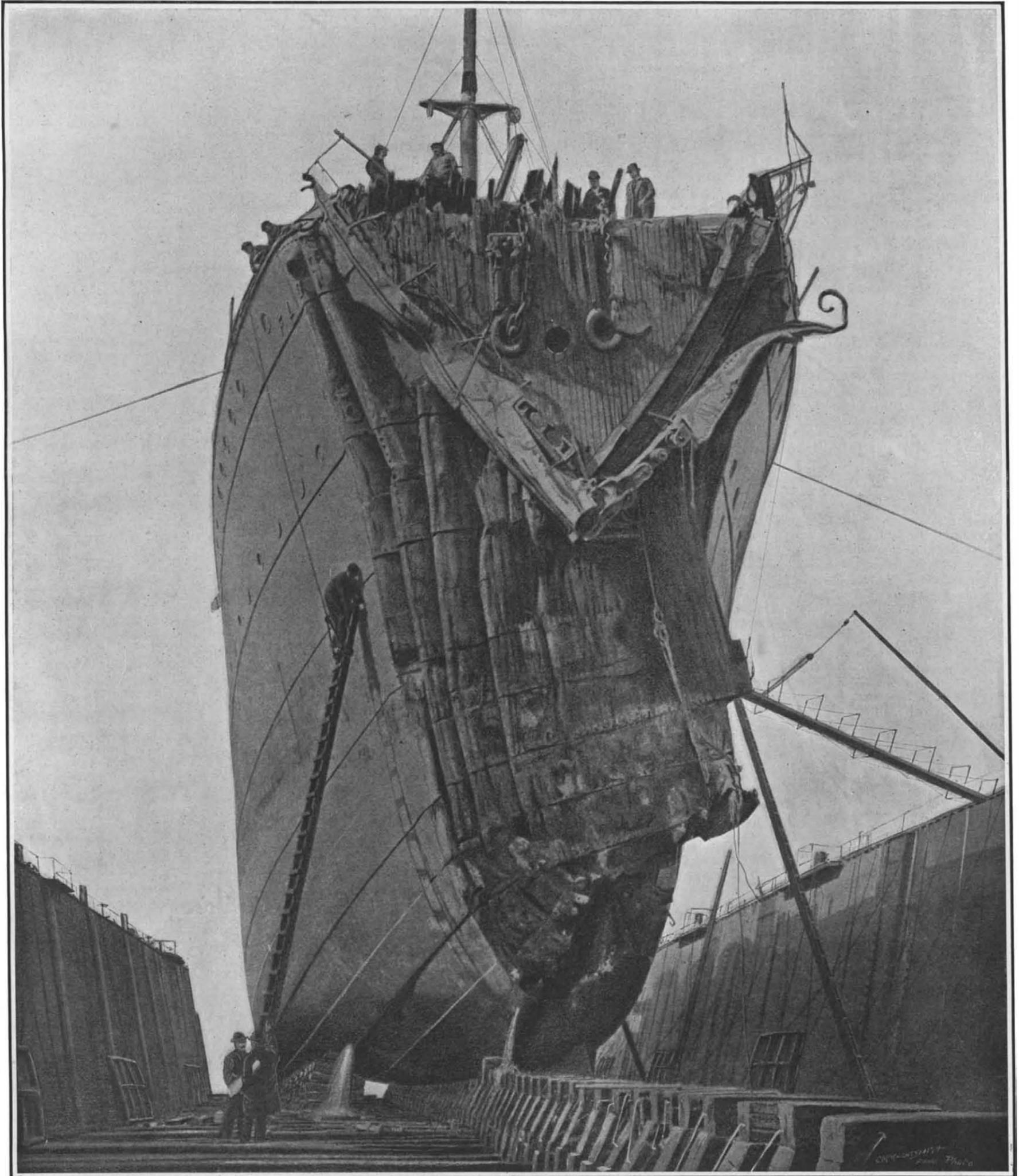
The above illustration shows the "Florida" in the Morse drydock for repairs. The force of the collision flattened thirty feet of the bow, concertina fashion, into a space of five feet. The wreckage was cut away and a new bow built on in twenty-four days.
