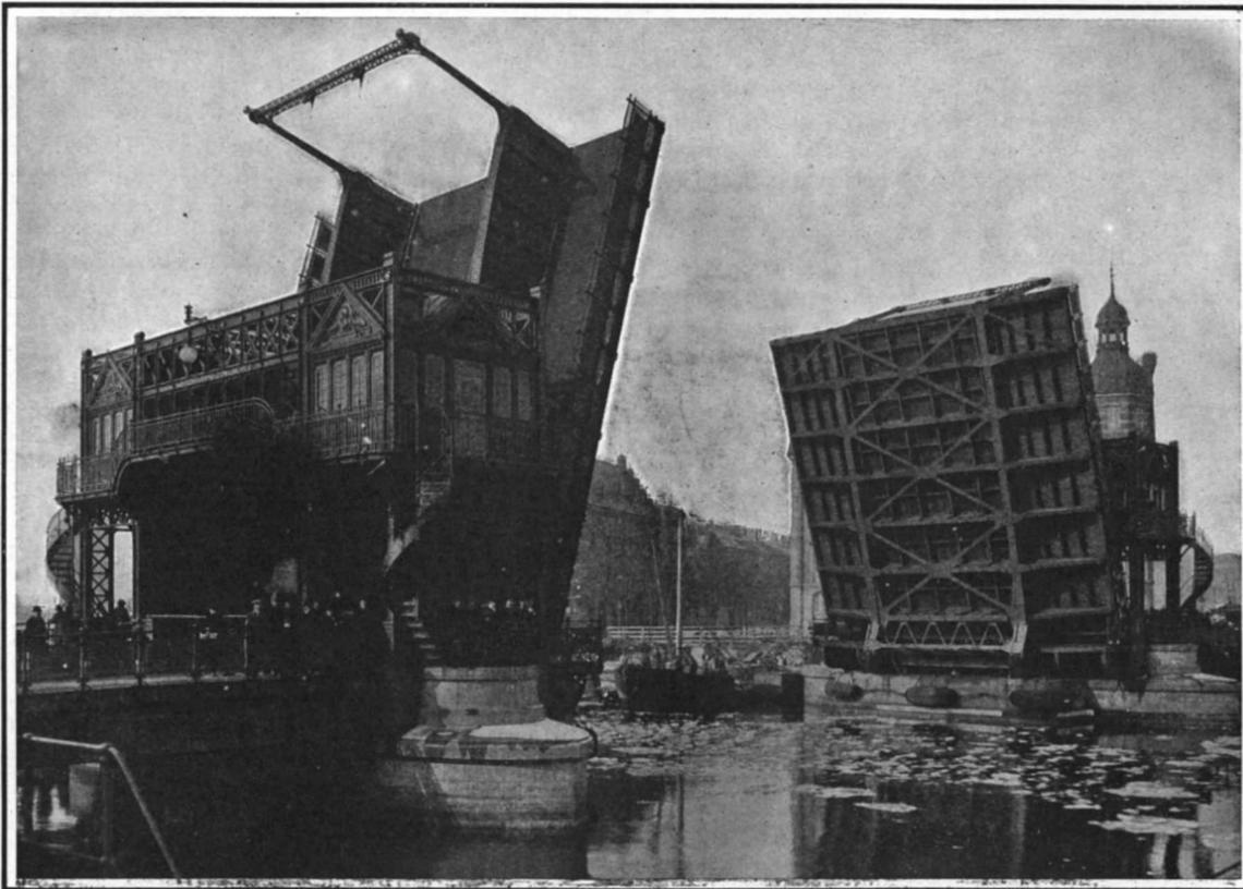
Width of opening, 92 feet 6 inches. Width of bridge roadway, 22 feet 7 inches. Width of each sidewalk, 10 feet 3 inches.
