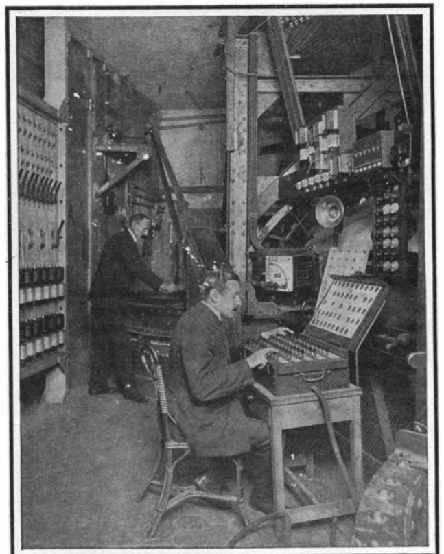
The keyboard by means of which the illumination is changed.
