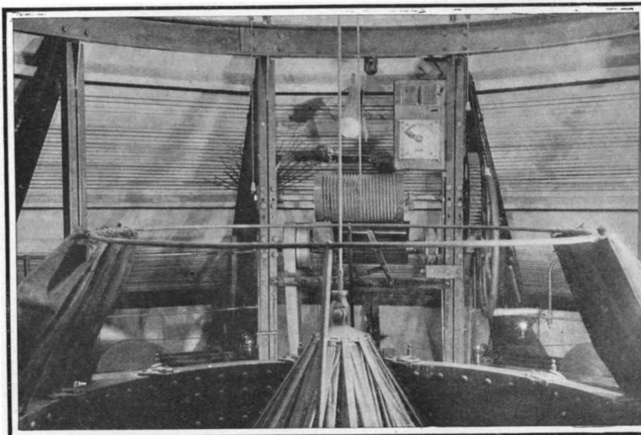
The mechanism by which the painted fabric is dropped which serves as the leafy roof of the central hall in the forest scene.
