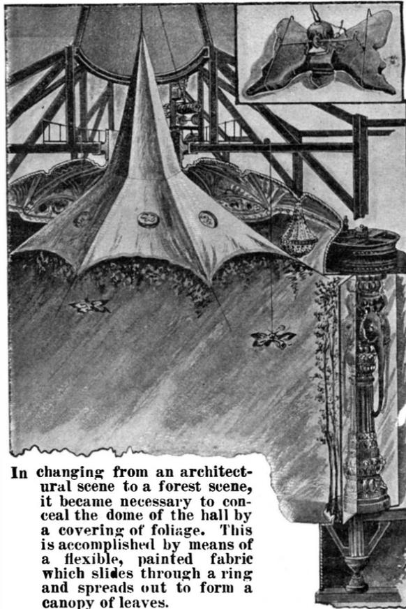
In changing from an architectural scene to a forest scene, it became necessary to conceal the dome of the hall by a covering of foliage. This is accomplished by means of a flexible, painted fabric which slides through a ring and spreads out to form a canopy of leaves.
