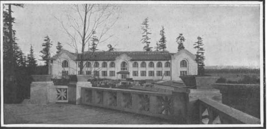
Machinery hall, one of the permanent structures.
