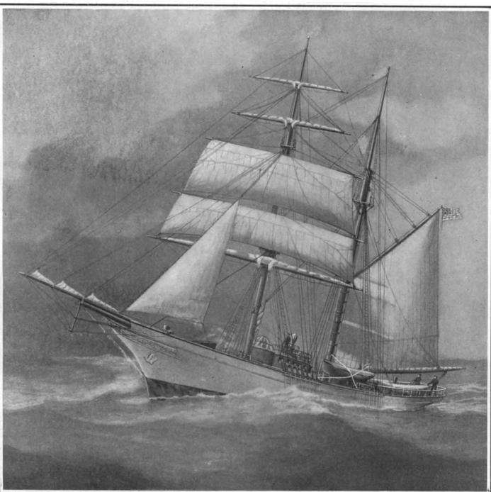
This interesting vessel is being built for the Carnegie Institution at Washington. Her survey of the oceans will form part of a comprehensive survey of the wnole world, on land and sea, by which the magnetic variation of the compass is to be determined. No iron, steel, or other magnetic material will be used in her construction.
