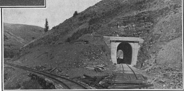
Relocation; the new line through the tunnel takes the place of the longer line around the hill. THE EXTENSION OF THE CHICAGO, MILWAUKEE & ST. PAUL RAILWAY TO THE PACIFIC COAST.
