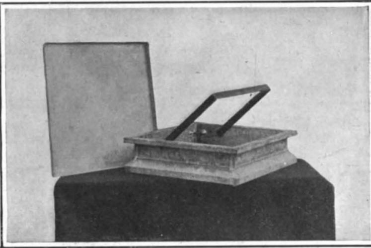
Fig. 7.—Reighard water glass for observation or photography of objects under water.
