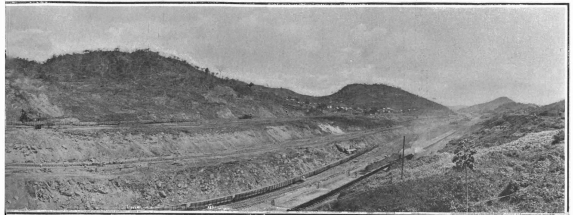
stretch between Gold Hill and Cucuracha is sliding, necessitating much extra excavation,
