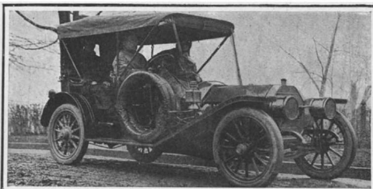
4-cylinder; cellular radiator; low-tension magneto ignition; selective sliding gear transmission; shaft drive.
