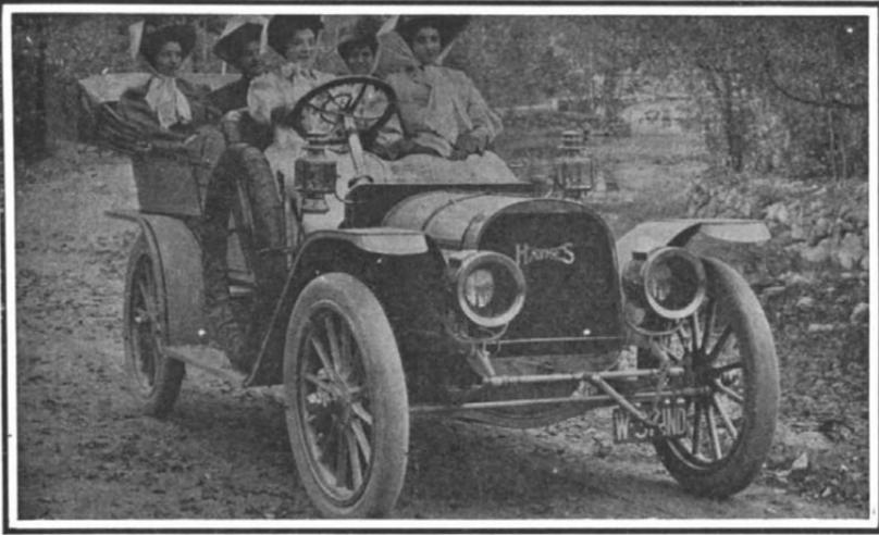
Wheel base, 112 inches; 36 horse-power; 4 cylinders, 4 1/4 x 5 inches; cellular radiator; dry battery and high-tension ignition; contracting band clutch; selective sliding gear transmission with three speeds forward and one reverse; shaft drive.
