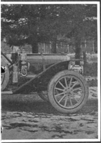
Under Rambler is a spare wheel, complete with tire. The regular wheel is screwed to the hub in three minutes.
