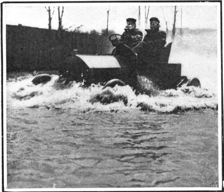
A waterproof Premier car running through water, even though the low-tension magneto is submerged.
