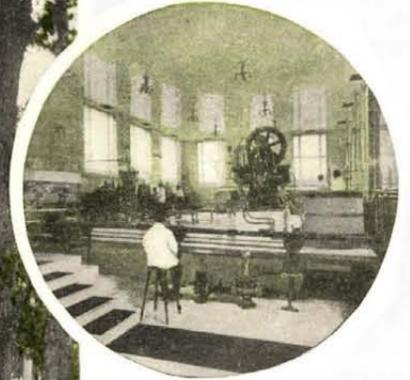
Poland Water Bottles may be seen in the foreground upon the conveyer belt, which has the capacity of carrying, each ten hours, fifteen thousand bottles between the washing, bottling and shipping rooms.
