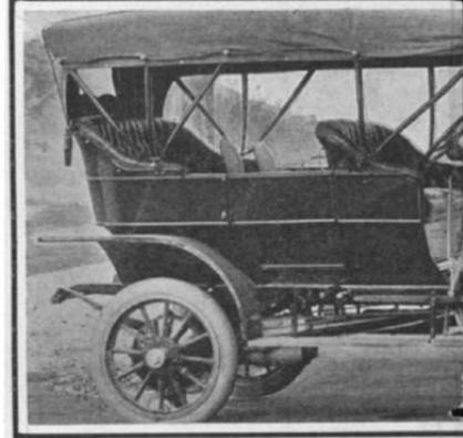
4 cylinders; 45 horse-power; speed, 8 to 50 miles unit coil; storage battery; high-tension magneto Selective sliding gear transmission. Thre
