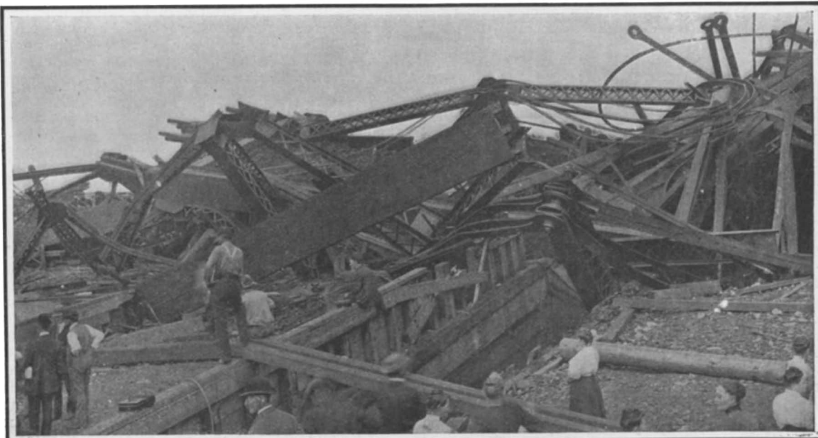
View of Wreck from Opposite Side to That Shown Above. FALL OF THE B. & O. SUSQUEHANNA BRIDGE.
