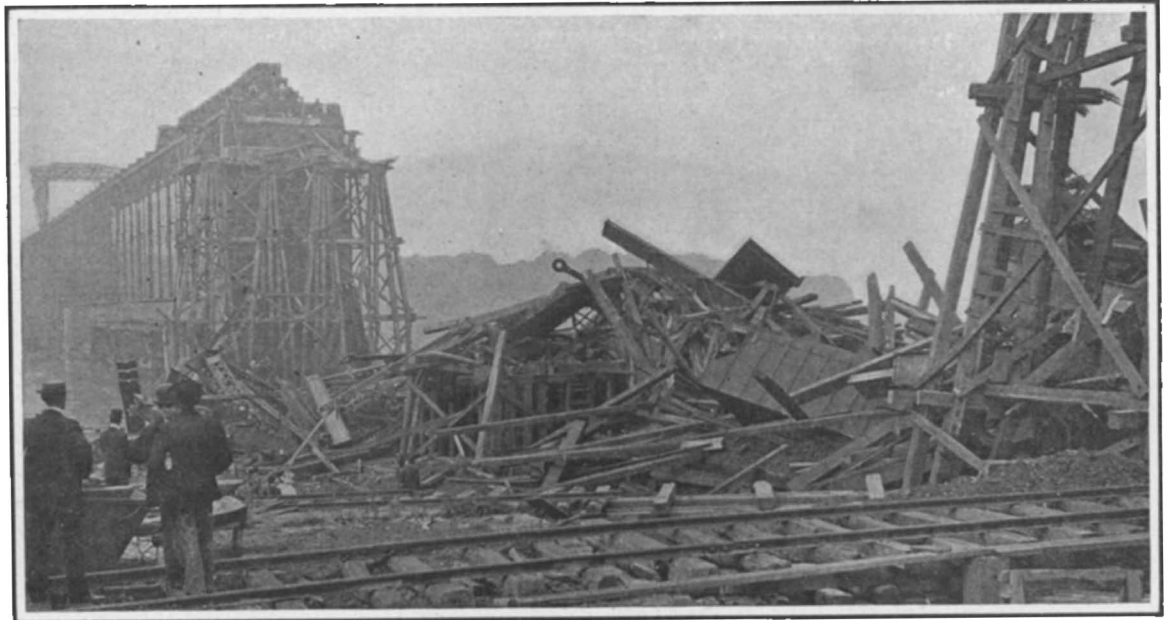
In This Wreck Are the Temporary 377-Foot Span, the Falsework, and 12 Loaded Coal Cars.
