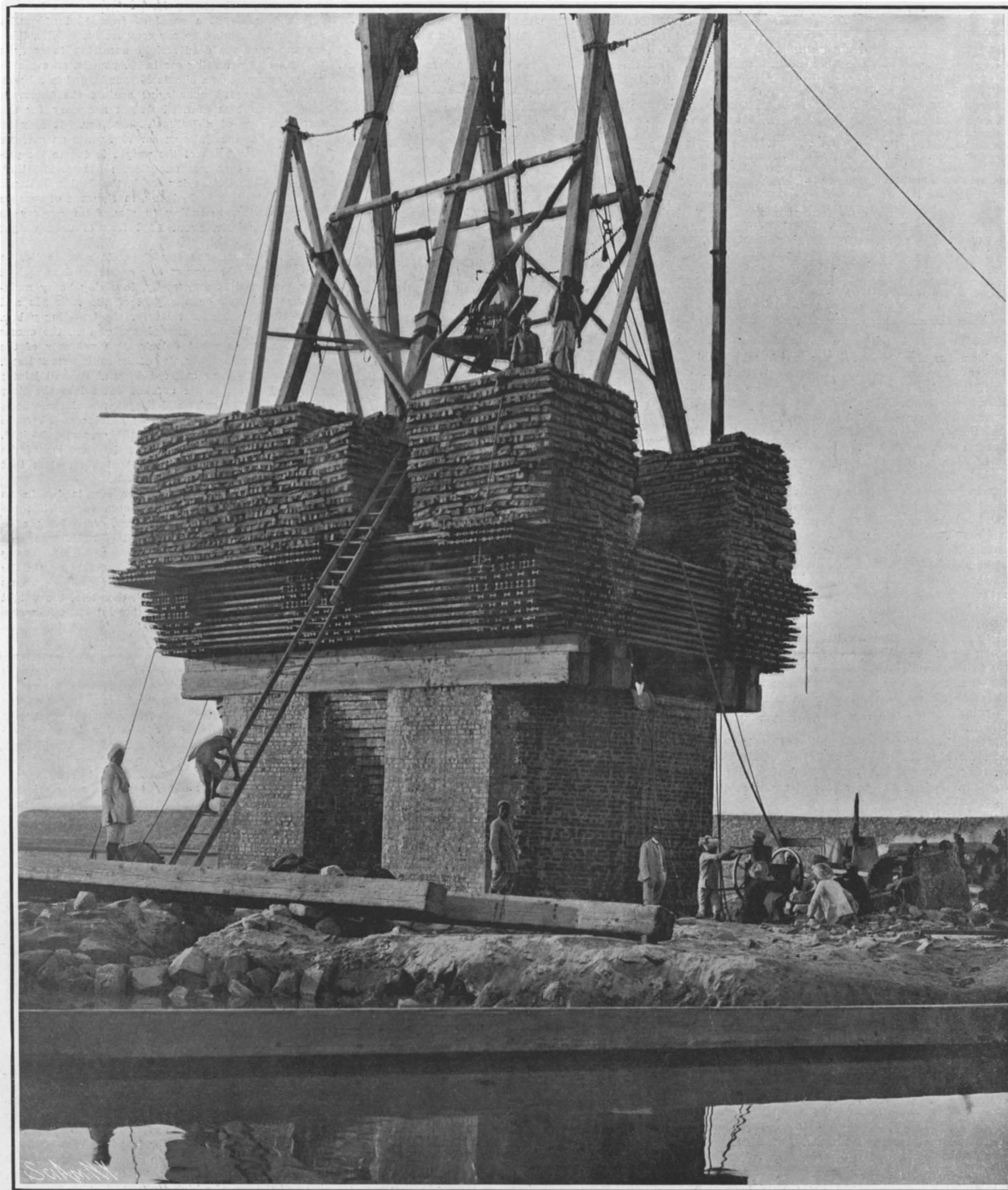
Brick Wells for the Pier Foundations Were Sunk Under an Artificial Load of Iron Rails, Pig Iron, and Sand Until Stanchied in a Substratum of Clay.
