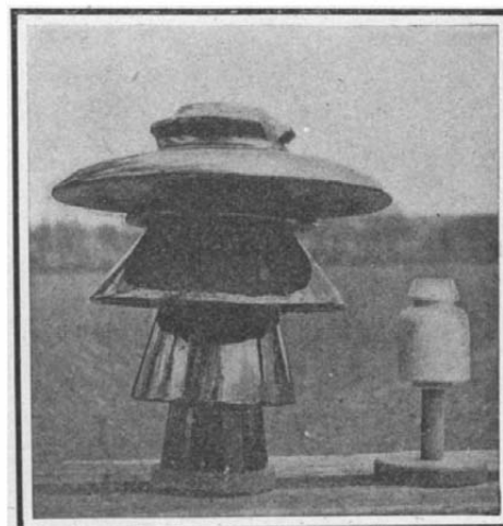
Insulator for Supporting Discharging Wire Compared with the Ordinary Telegraph Insulator.
