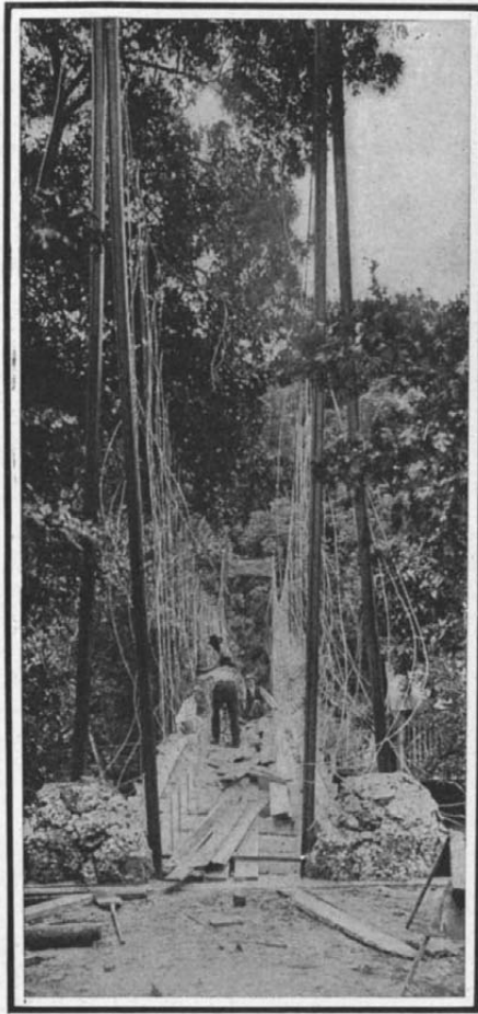
The Bridge as Viewed from the North Bank. Note the Steel Rail Towers.
