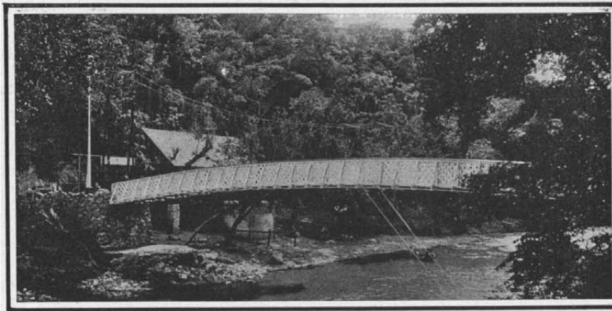
The Completed Suspension Foot Bridge across Rock Creek, Platt National Park.
