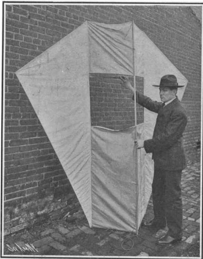
King Kite Used for Raising Antennæ Wire.
