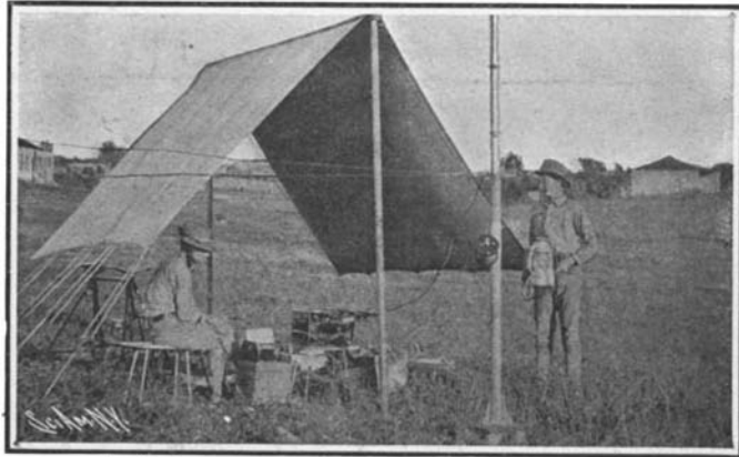
Portable Wireless Telegraph Station in Use in Cuba.
