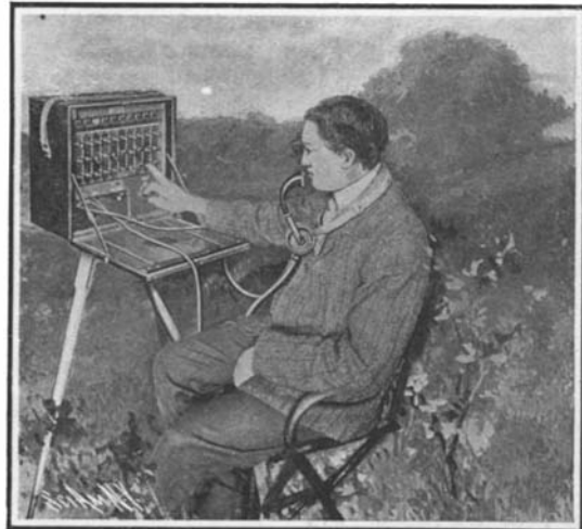
Portable Field Telephone Switchboard.
