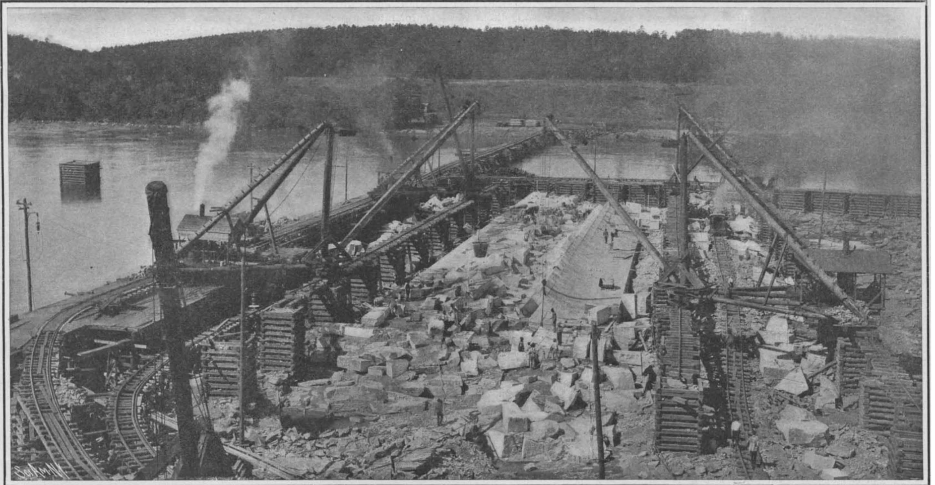
The Cofferdam and Commencement of the Permanent Work.
