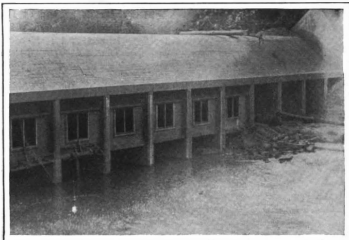
Downstream View of Dam, Showing Windows for Lighting the Power Chamber.
