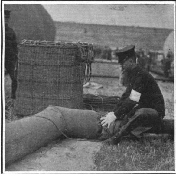
The Connection Between the Balloon and the Gas Main.
