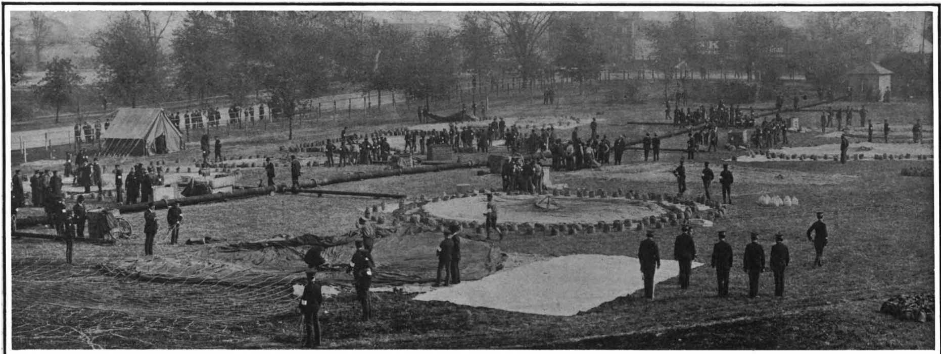
View of the Park Before the Balloons Were Inflated. The Gas Mains Connected and the Ballast Bags Ready.
