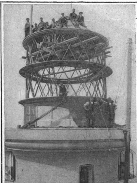
The Lantern in Course of Construction.
