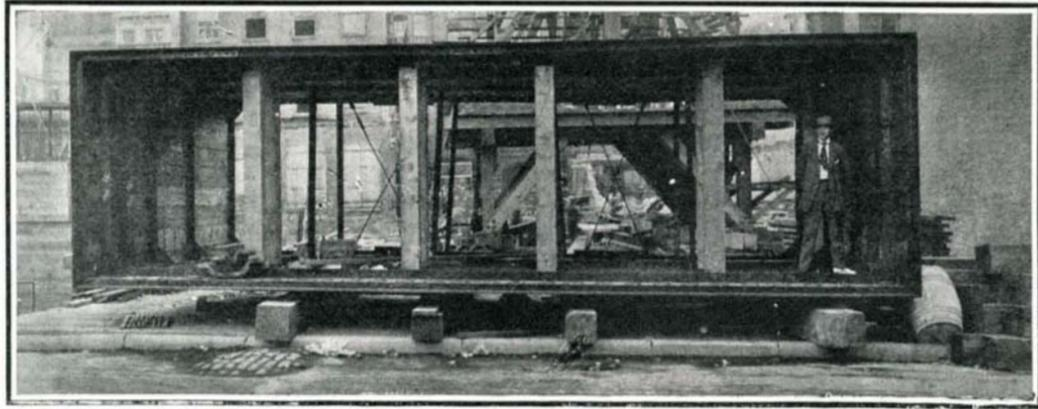
One of the Caisson Forms Used in Building and Sinking the Huge Concrete Wall, 8 Feet Thick and 75 Feet Deep, Inclosing the Foundations of the Cortlandt Street Terminal Station.
