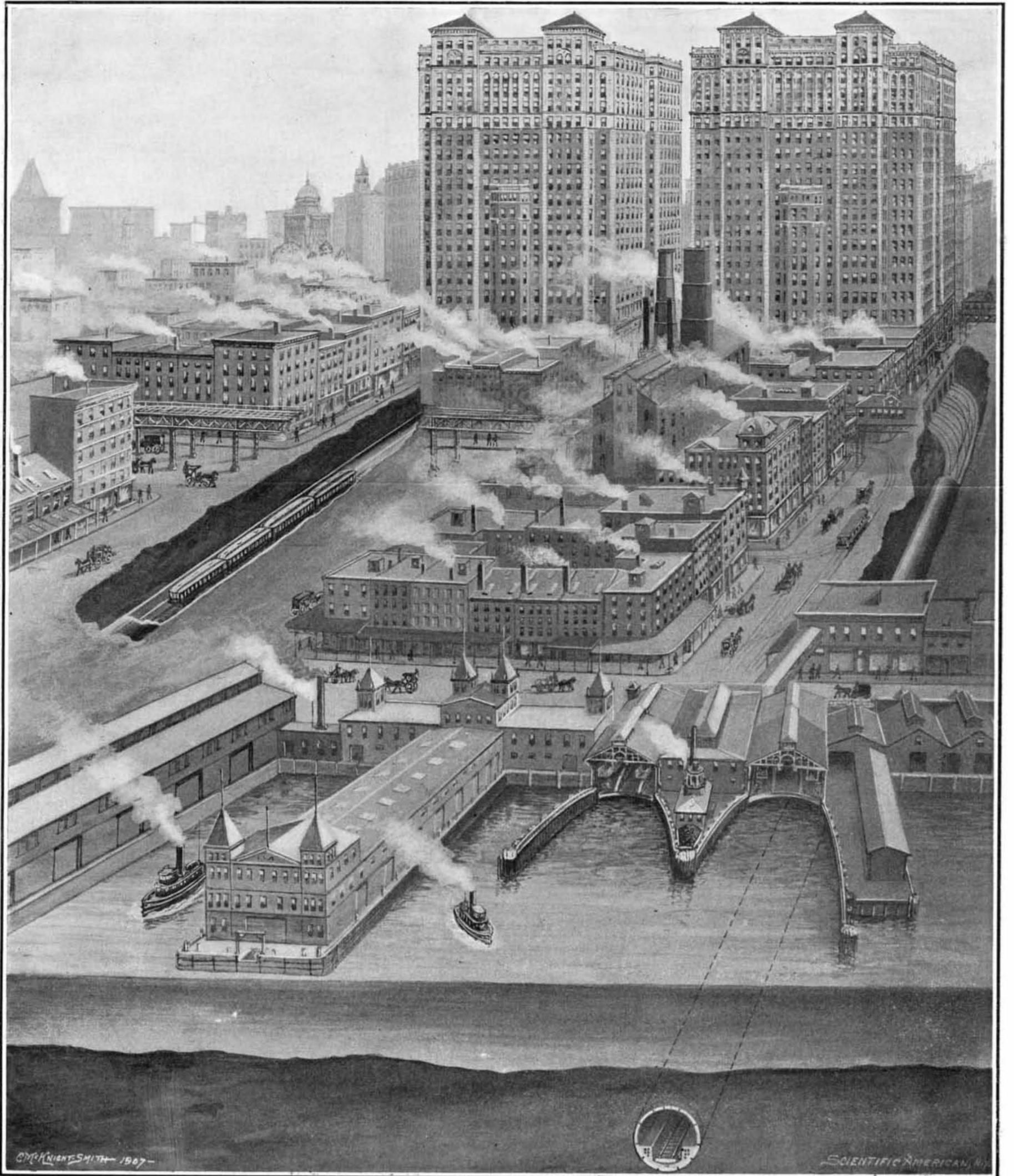
The trains from Jersey City will enter Manhattan by the tube shown in the foreground. The single track will diverge into five tracks, which will swing to the left and enter a six-platform station below the large building shown in the background. This building, 22 stories high, will be nearly three times larger than any existing office building and will house 20,000 people. Trains return to Jersey City by the tunnel shown at the left of building.
