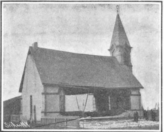
The Walls Blown Out.
