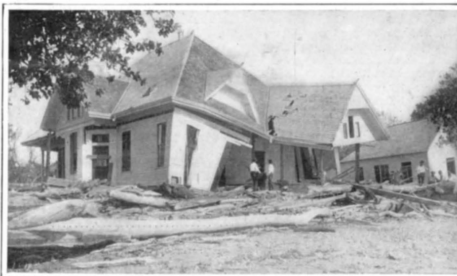
A House on the Long Shell Road; the Collapse Was Due to the Washing Away of the Foundations.
