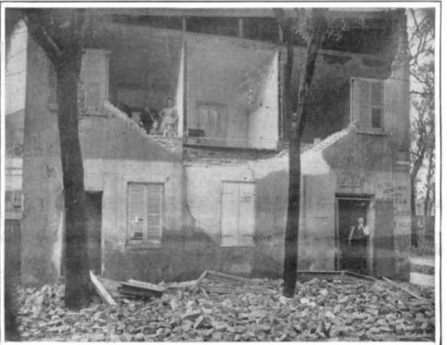
House on St. Louis Street With a Side Blown Away.
