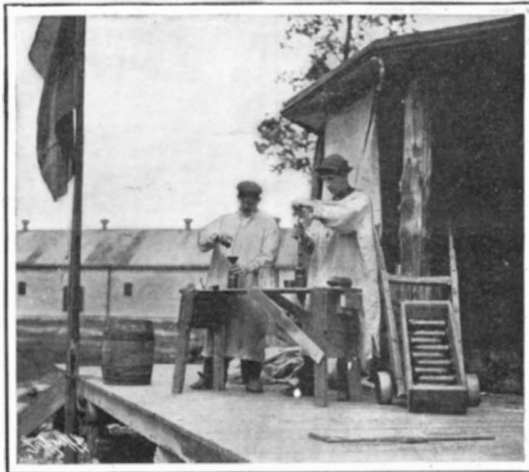
One of the Powder Filling Houses Charging 3-Inch Shells.
