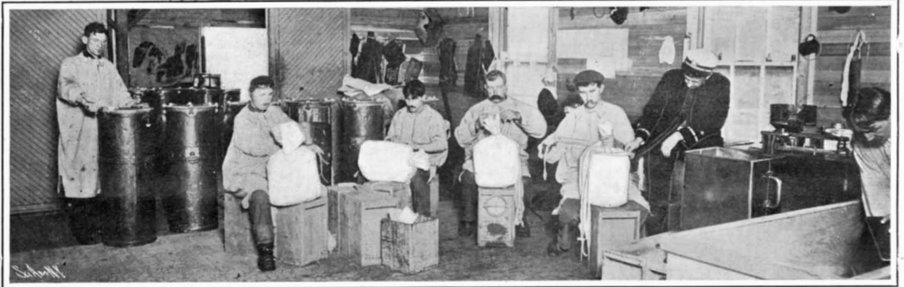
Interior of the Main Powder Filling House, Iona Island, Where the Smokeless Powder is Put Up in Bags Which Constitute the Firing Charges of Naval Ordnance.
