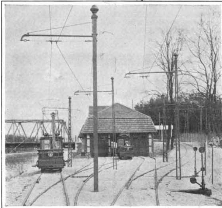
The Switches Near the Locomotive Shed.
