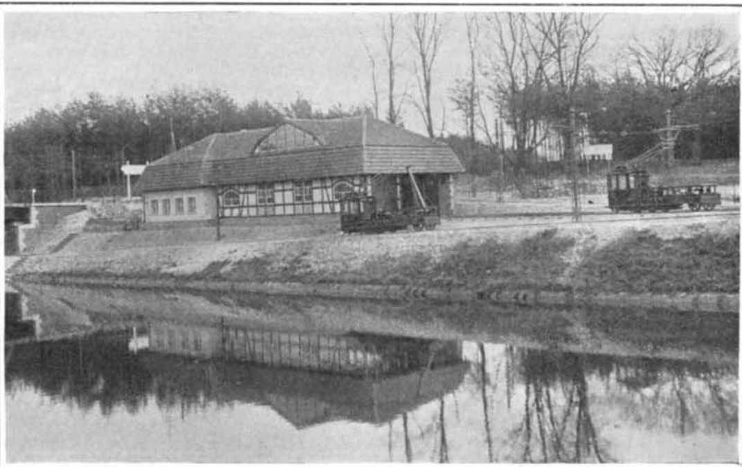
Shed for Electric Towing Locomotives
