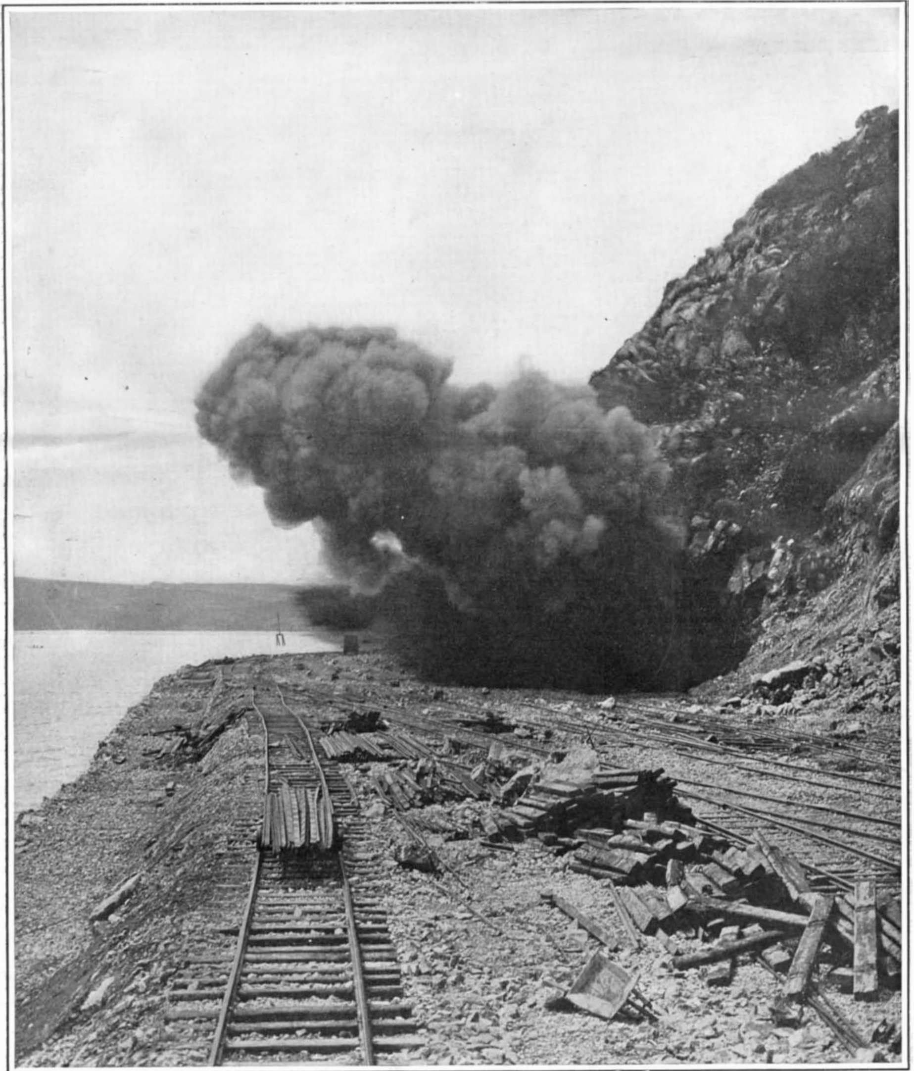
BLASTING AT FISHGUARD, WALES, FOR THE NEW ROUTE FROM ENGLAND TO IRELAND.—[See page 262.]
