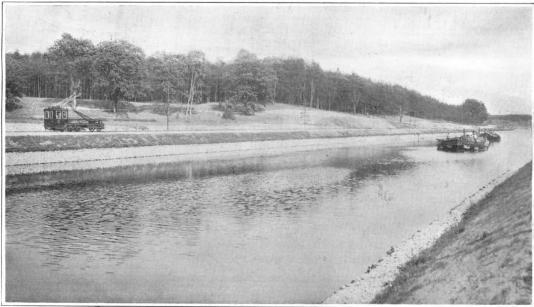
Towing Barges by Electric Locomotives on the Teltow Canal.
