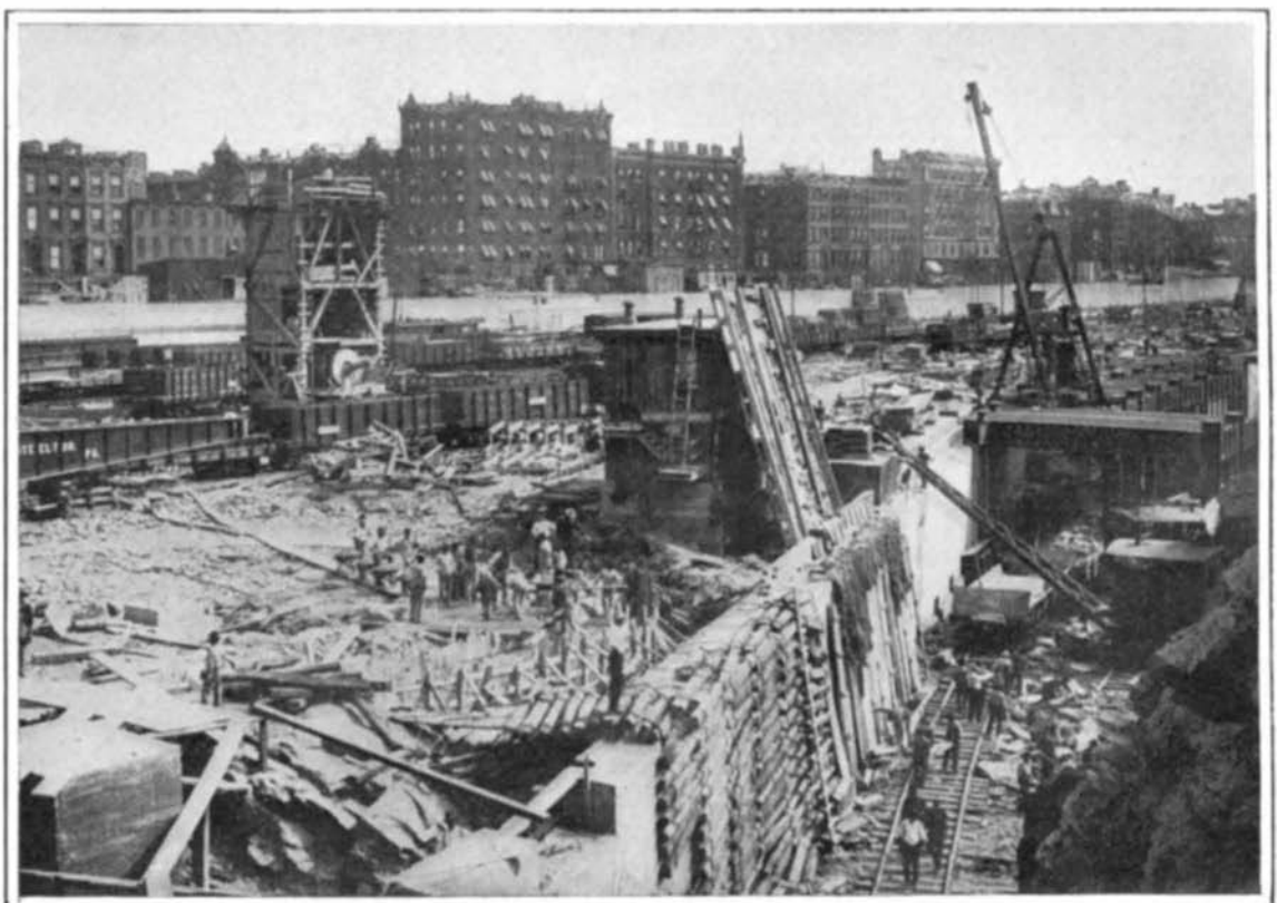
View of Excavated Easterly Portion of Grand Central Yard Looking South, Showing Suburban Level and Steelwork for Carrying Upper Express Level. The Retaining Wall to the Left Fronts on Lexington Avenue.
