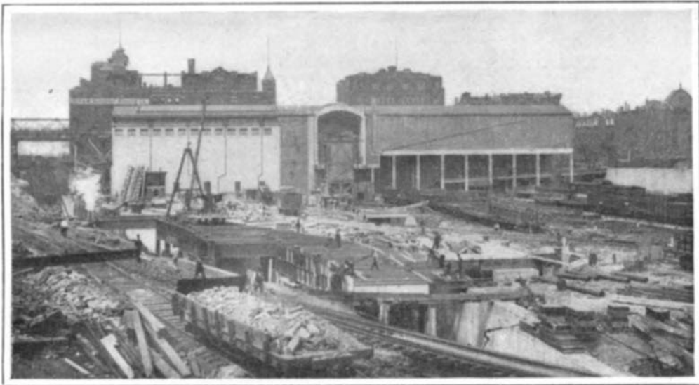
Northeasterly Portion of Grand Central Yard, Showing Sub-station, Express Level, and Steelwork Erected Above Suburban Level.
