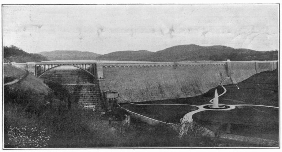
Total length dam and spillway, 2,168 feet. Height, foundation to crest, 297 feet. Width at base of foundations, 216 feet. Depth of foundations, 140 feet. Storage capacity, 30,000,000,000 gallons. Cost, \$7,631,189.
