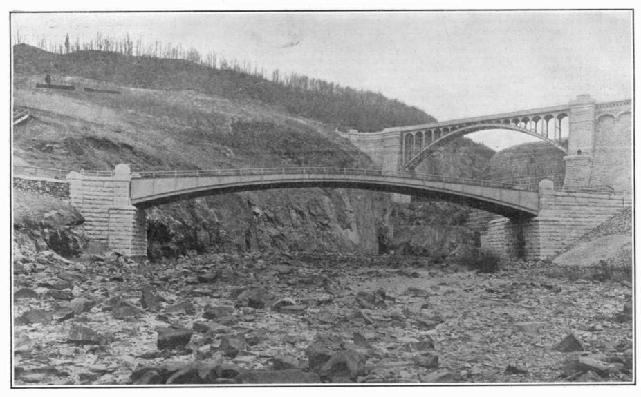
The upper bridge is 200 feet and the lower bridge 150 feet in length.
