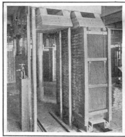
Fig. 11.—Pressing 5,000 Bunches for Cheroots in Molds at One Time in 30 Seconds.
