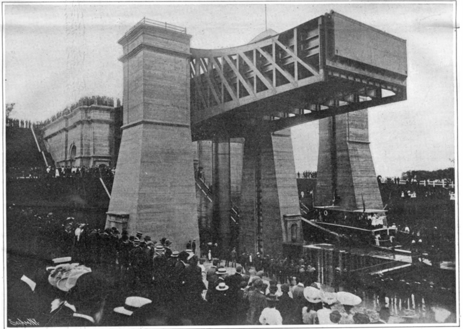
View on the Opening Day. The West Chamber is Elevated to Full Height. The East Chamber Contains a Steamer About to be Raised.
