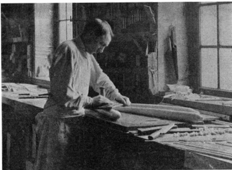
Fig. 5.—Rolling Wax Candles.
