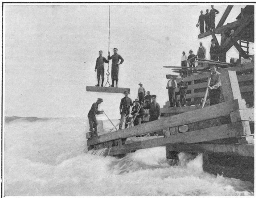
Launching a crib in 26 feet of water in the upper rapids where the water is running at 15 miles an hour.
