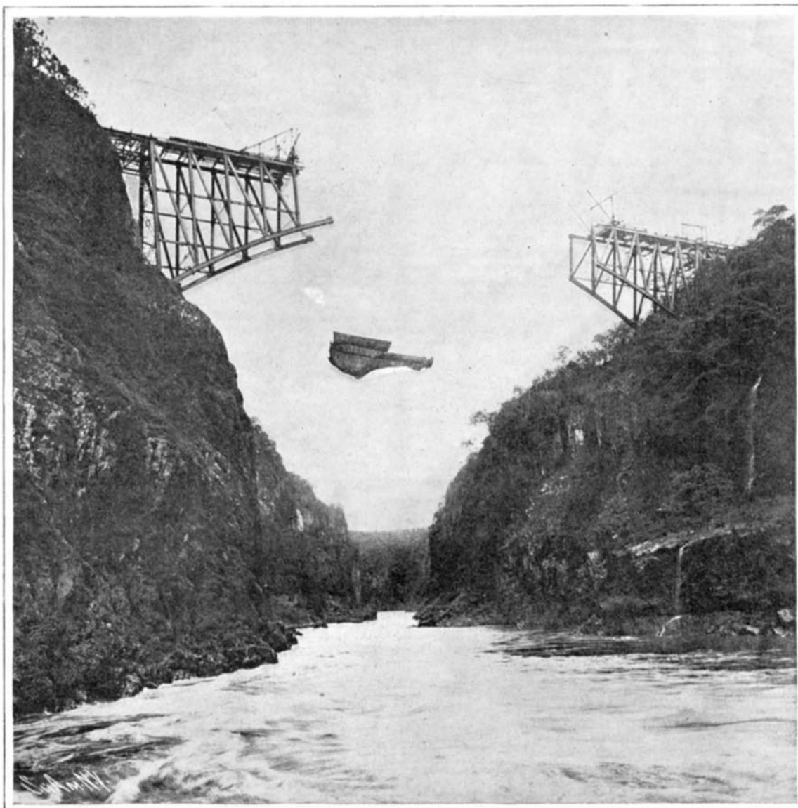
THE VICTORIA FALLS BRIDGE IN COURSE OF ERECTION. THE MATERIAL WAS CARRIED BY CABLEWAY.
