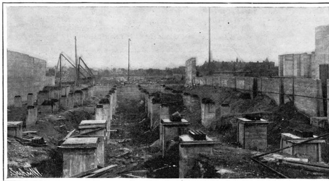
Columns Supporting the Interior Structure.
