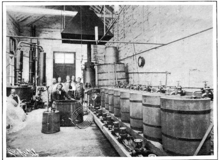
At the right: Exhauster for extracting sugar formed in digester. At the left: Alcohol stills.
