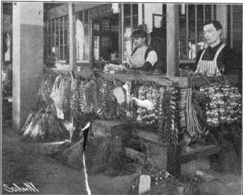
Wiring Articles for Plating.
