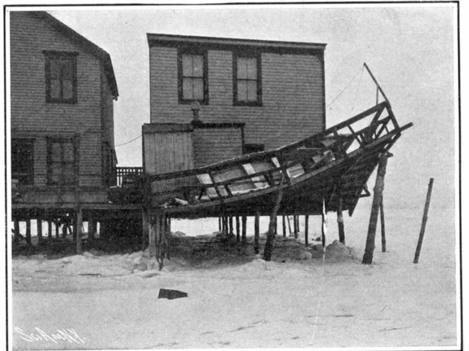
THE UPLIFTING OF BUILDING FOUNDATIONS BY ICE IN JAMAICA BAY, NEW YORK.
