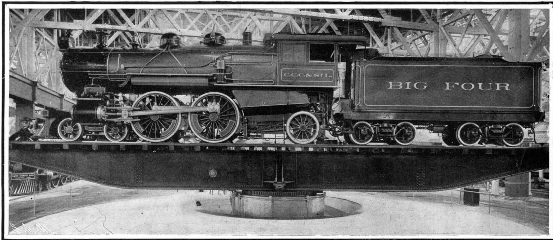
Engine and Tender weigh 163 tons. The turntable is 70 feet long by 5 feet deep.
