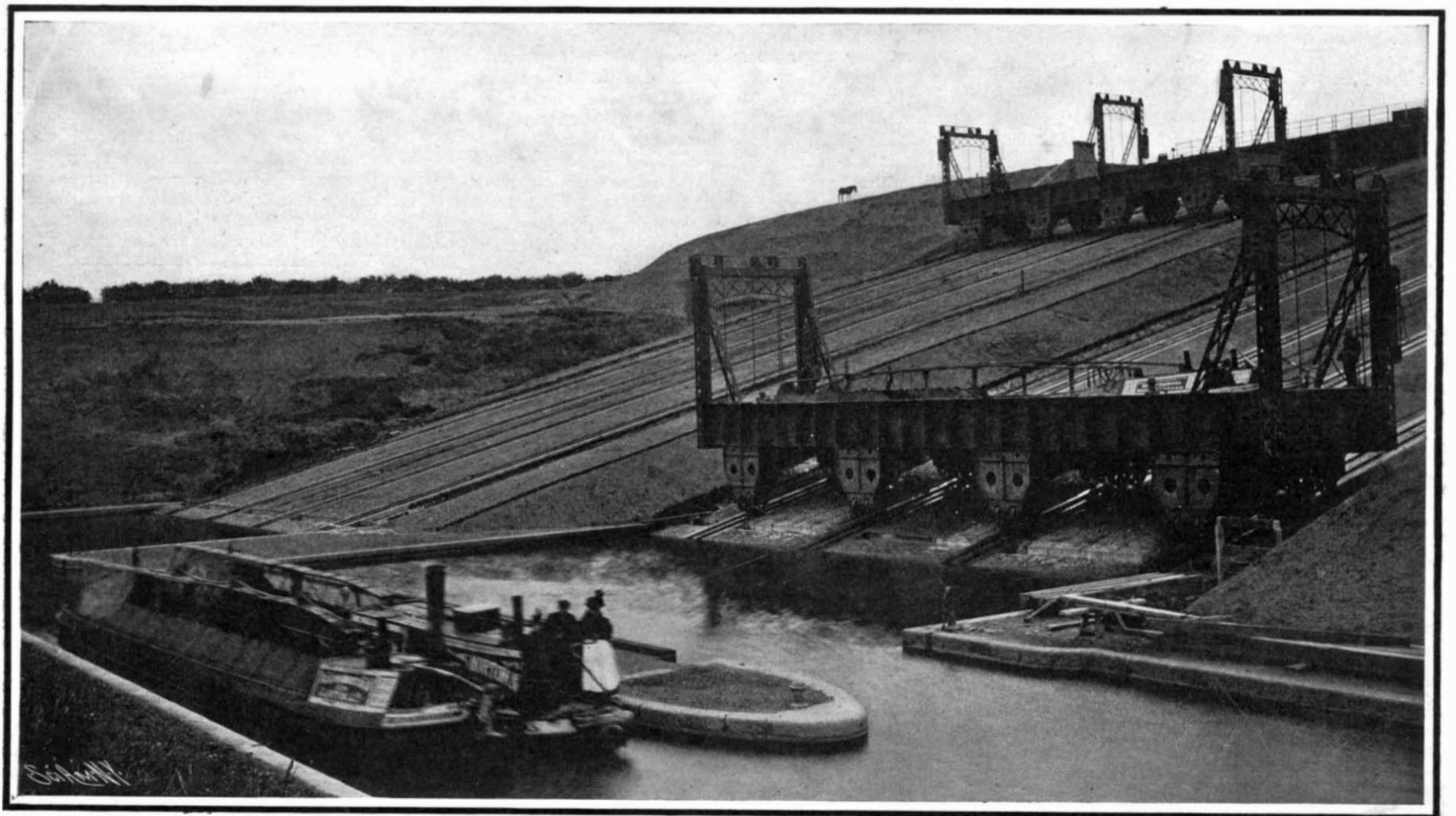
The Barge Lift in Operation. Descending Tank Loaded. Height of Lift, 75 feet; Grade, 1 in 4.
