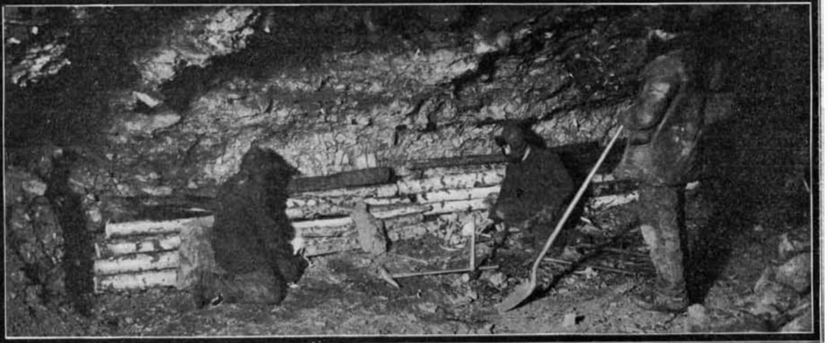
"Burning-in" with a Wood Fire.
