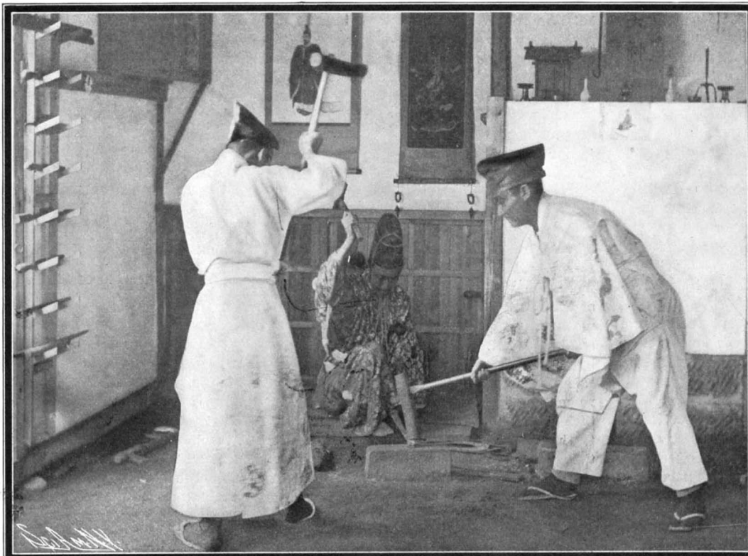
Forging One of the Ingots From Which the Sword is Made.
