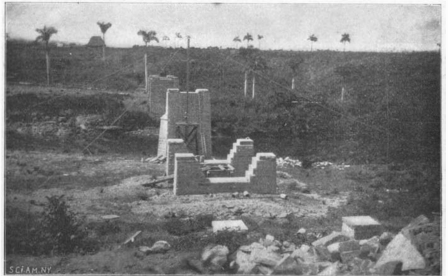
Masonry Piers for Bridge Across Guanimum River.
