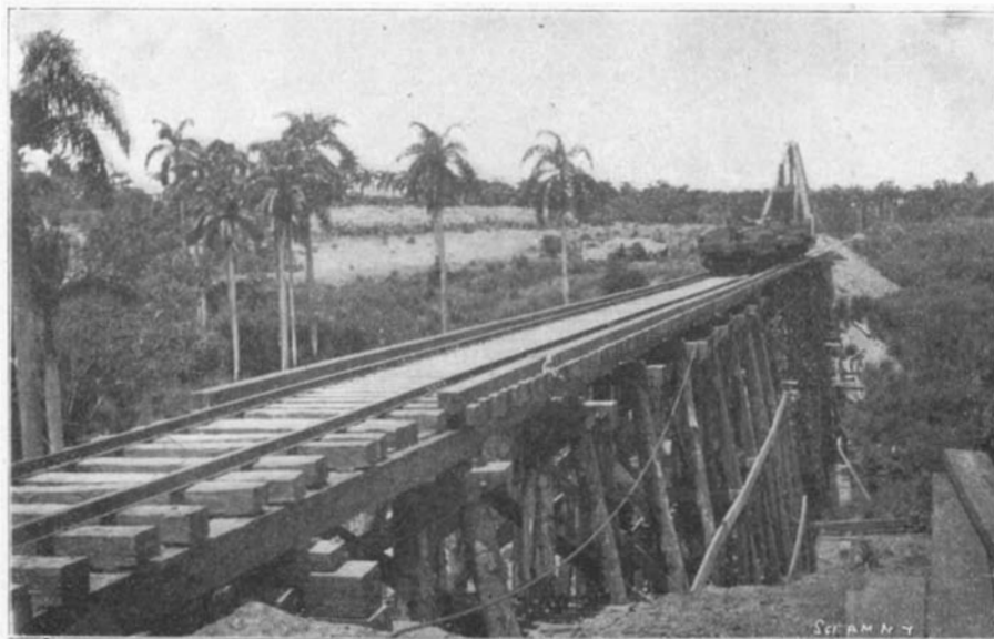
Pile Trestle Bridge on the Eastern Division.
