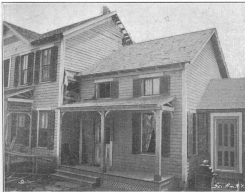
EFFECTS OF LIGHTNING, SHOWING WHERE THE BOLT ENTERED AT THE ROOF AND WHERE IT LEFT THE HOUSE AT THE SIDE.
