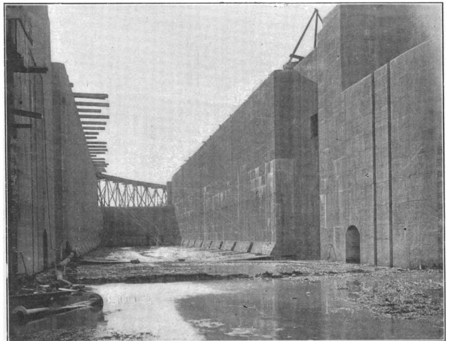
VIEW TAKEN IN INTERIOR OF ONE OF THE LOCKS.
