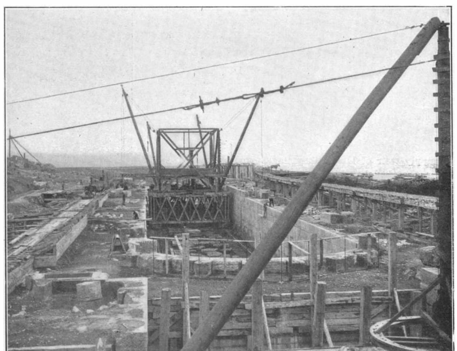
LOCK UNDER CONSTRUCTION—MASONRY PLACED IN POSITION BY DERRICK TRAVELING ON FLOOR OF DOCK.
