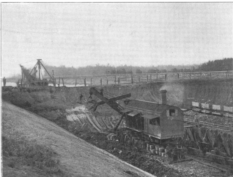
STEAM SHOVEL AND FLOATING DREDGE AT WORK ON CANAL.
