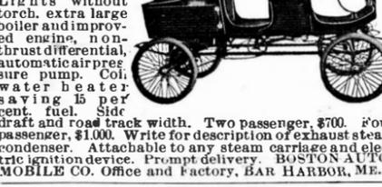
Latest and best steam carriage built. Following improvements: Lights without torch, extra large boiler and improved engine, non-thrust differential, automatic air pressure pump, coil water heater, saving 15 per cent. fuel. Side draft and road track width. Two passenger, \$700. Four passenger, \$1,000. Write for description of exhaust steam condenser. Attachable to any steam carriage and electric ignition device. Prompt delivery. BOSTON AUTO-MOBILE CO. Office and Factory, BAR HARBOR, ME.
