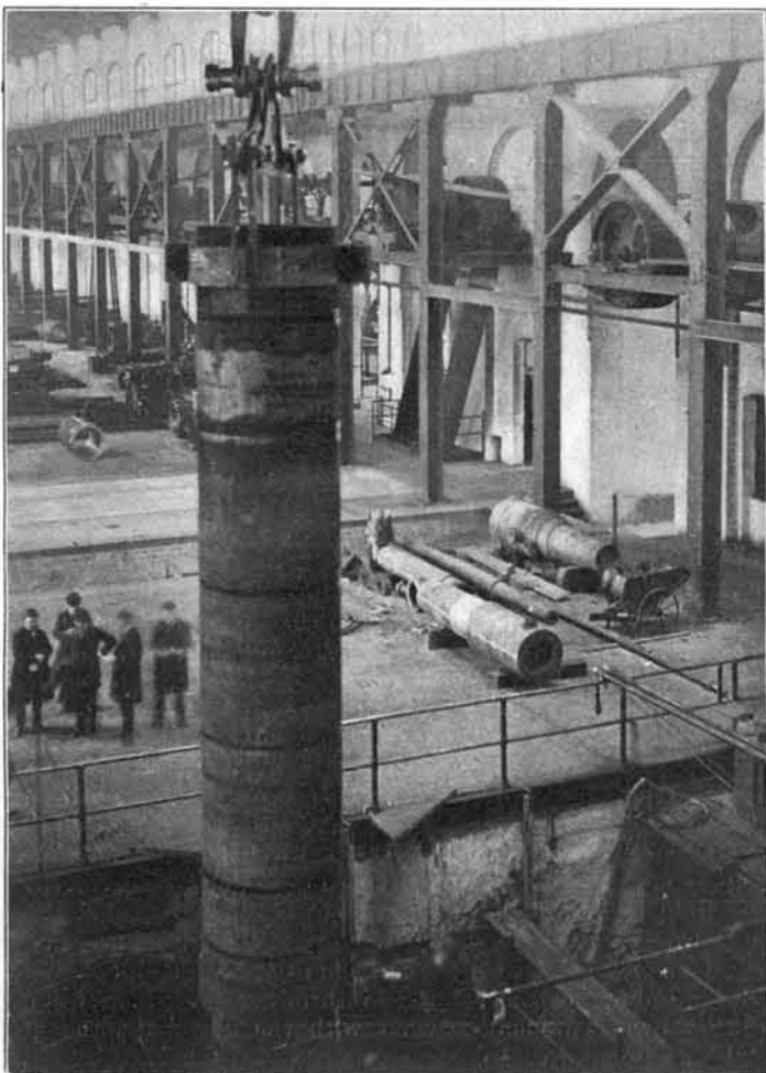
JACKET BEING REMOVED FROM THE SHRINKAGE FURNACE.
