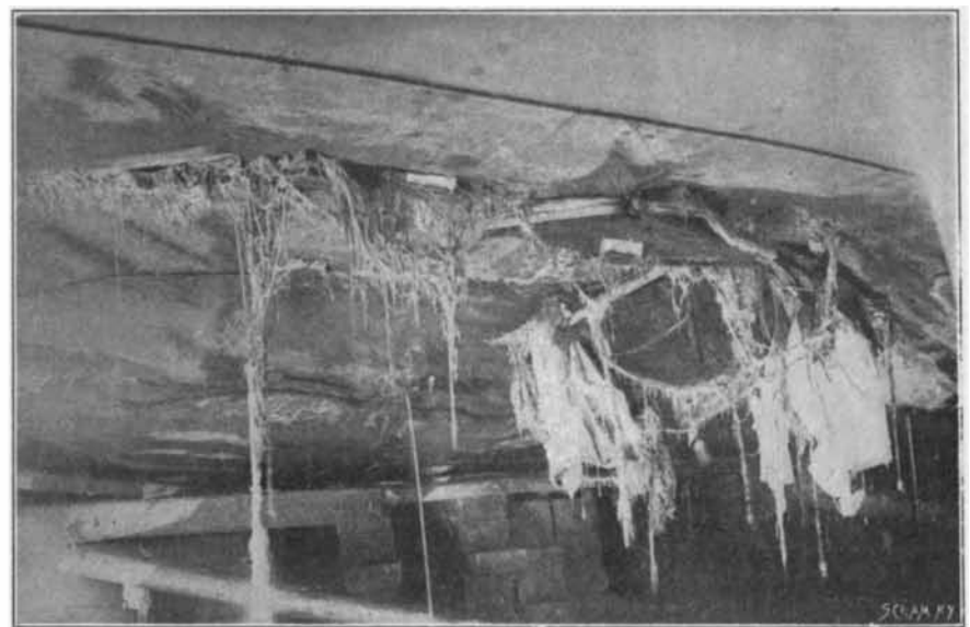
View from Port, Showing Temporary Patches Put on by Diver over Injuries between Frames 19 and 24.
