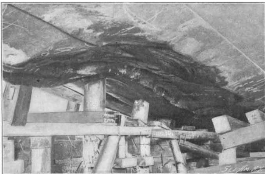
View from Port and Underneath, Showing Injury to Keel between Frames 14 and 19. Kure, July 25, 1900.
