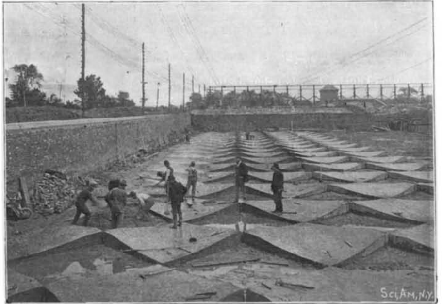
Placing the Groined Concrete Floor of a Filter.
