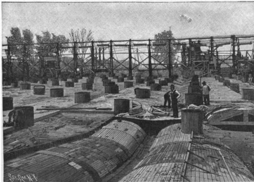
Constructing the Vaulted Roof of Filter.
