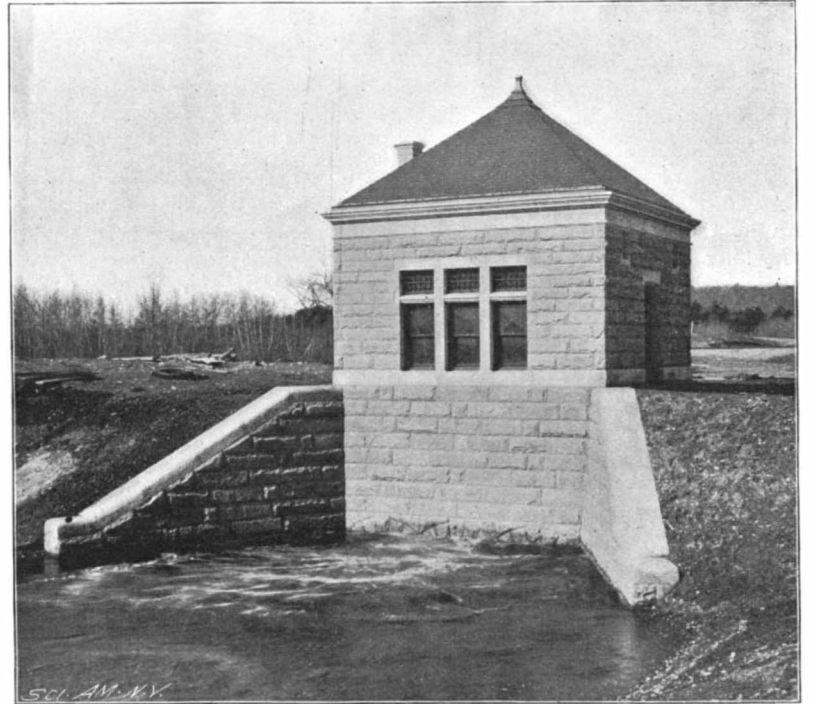
TERMINAL CHAMBER, WACHUSETT AQUEDUCT.
