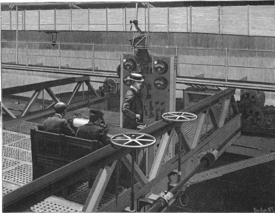
Fig. 6. Towing Carriage with Observers at Work.
