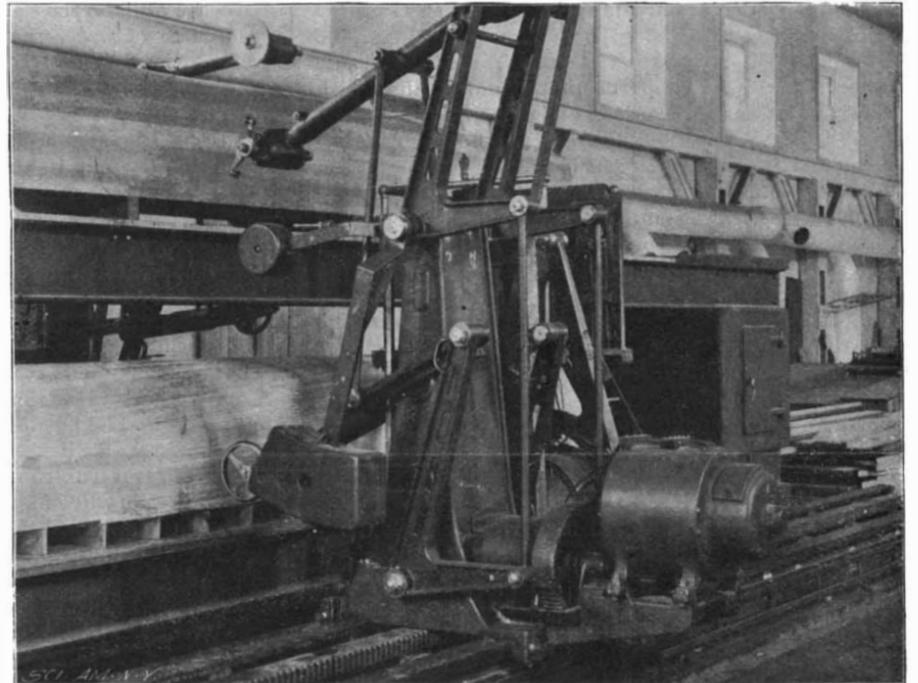
Fig. 4.—Model-Cutting Machine. ("Former" is Below, Model Above.)
