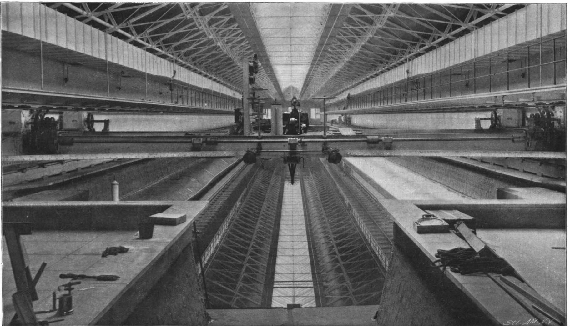
Fig. 5.—Interior View Showing Basin and Towing Carriage.
