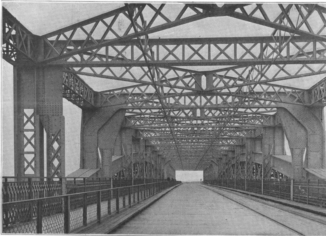
ROADWAY AND OVERHEAD WIND TRUSS OF THE LEVENSAU BRIDGE.
