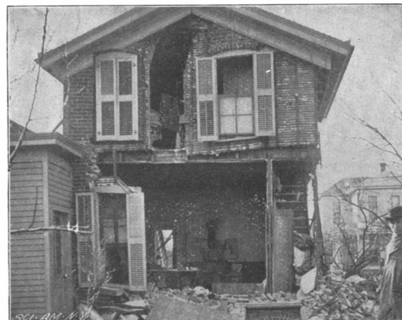
REAR OF HOUSE WRECKED BY GAS EXPLOSION.
