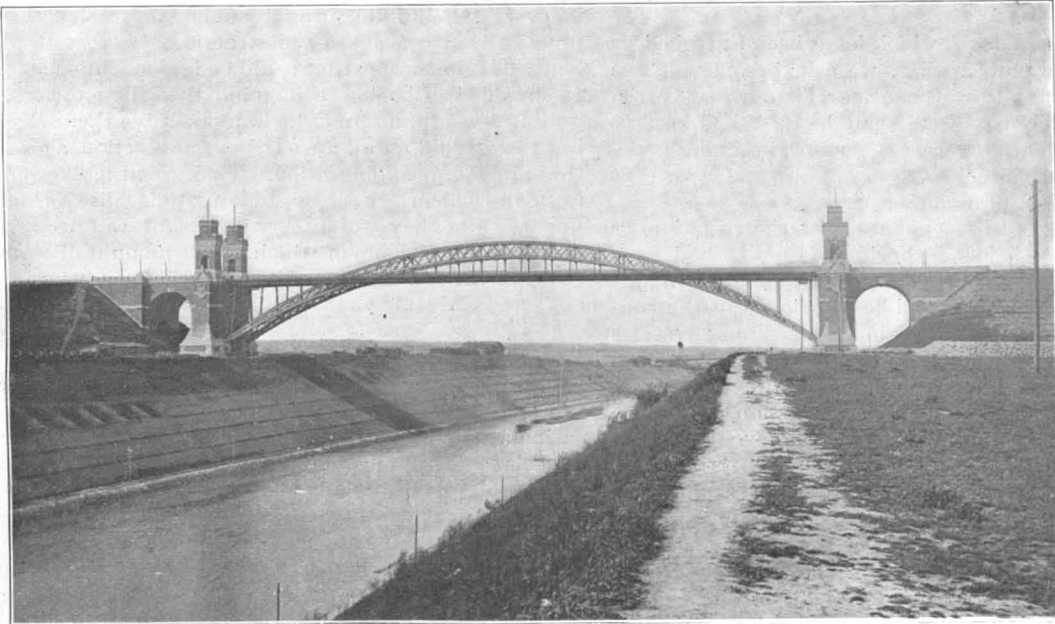
Grunenthal Bridge Across the Kiel Canal. Span, 511.7 Feet.
