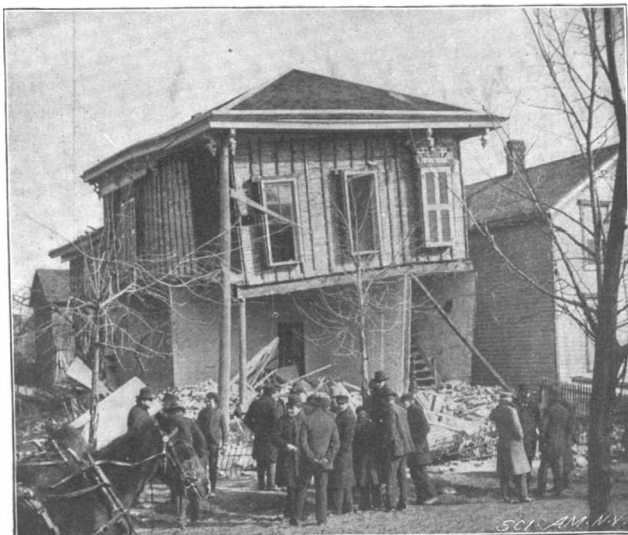
FRONT OF HOUSE WRECKED BY GAS EXPLOSION.
