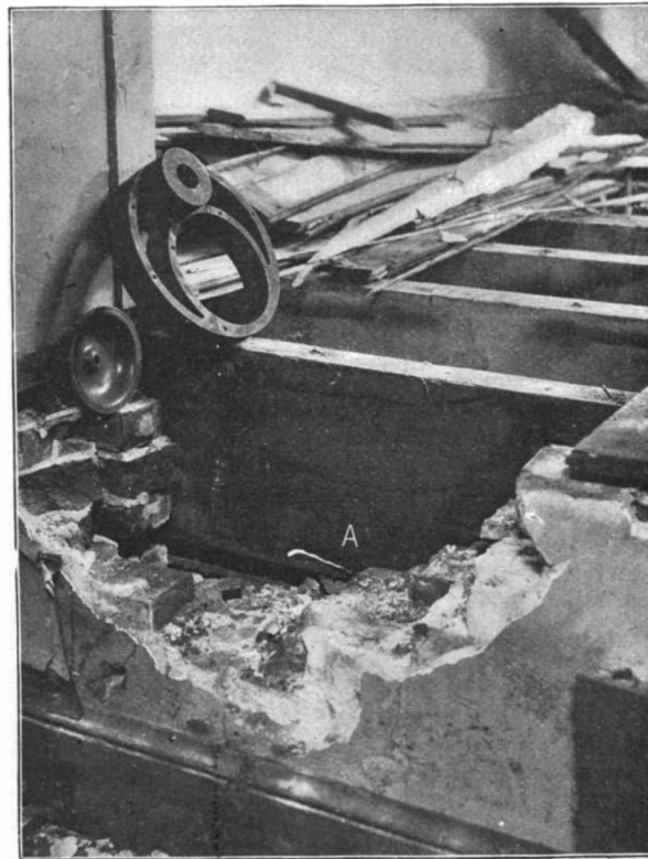
Threshold of Rear Exhibition Room, Showing Concealed Tube, A.
