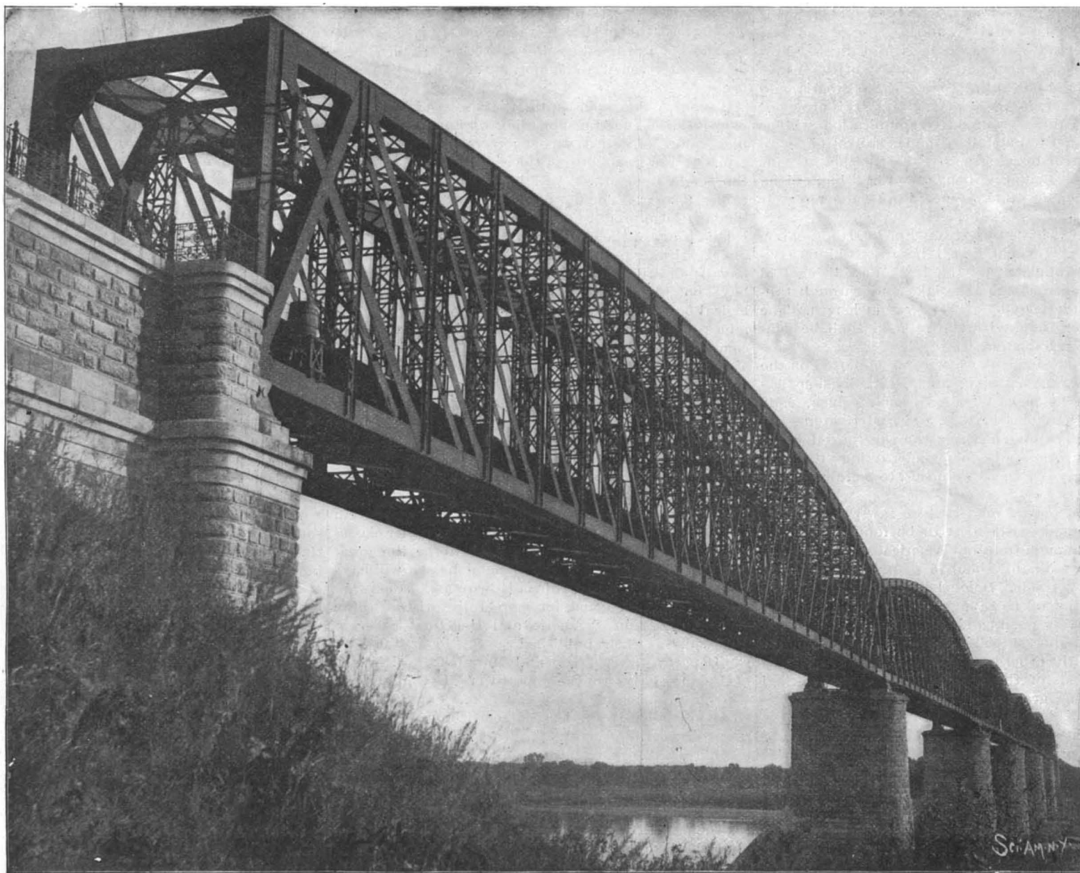
TRANSIBERIAN RAILWAY—STEEL BRIDGE AT OUFÀ, OVER THE BIELAIA RIVER.
