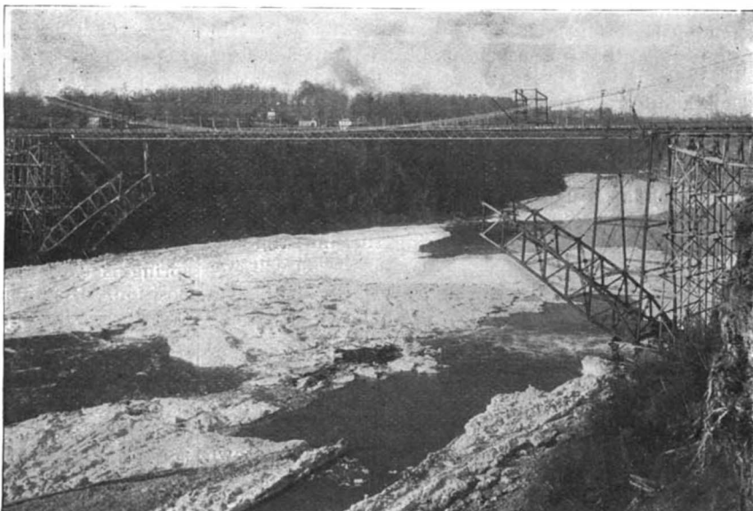
ERECTING THE STEEL ARCH WITH THE AID OF THE PRESENT SUSPENSION BRIDGE.
