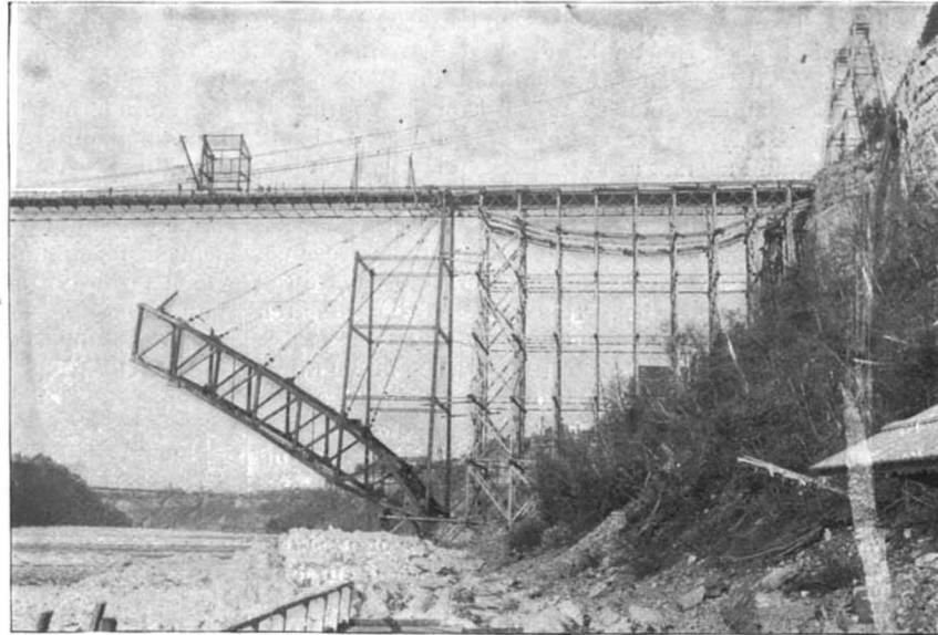
NIAGARA STEEL ARCH—FALSE WORK AND STEEL GUYS.
