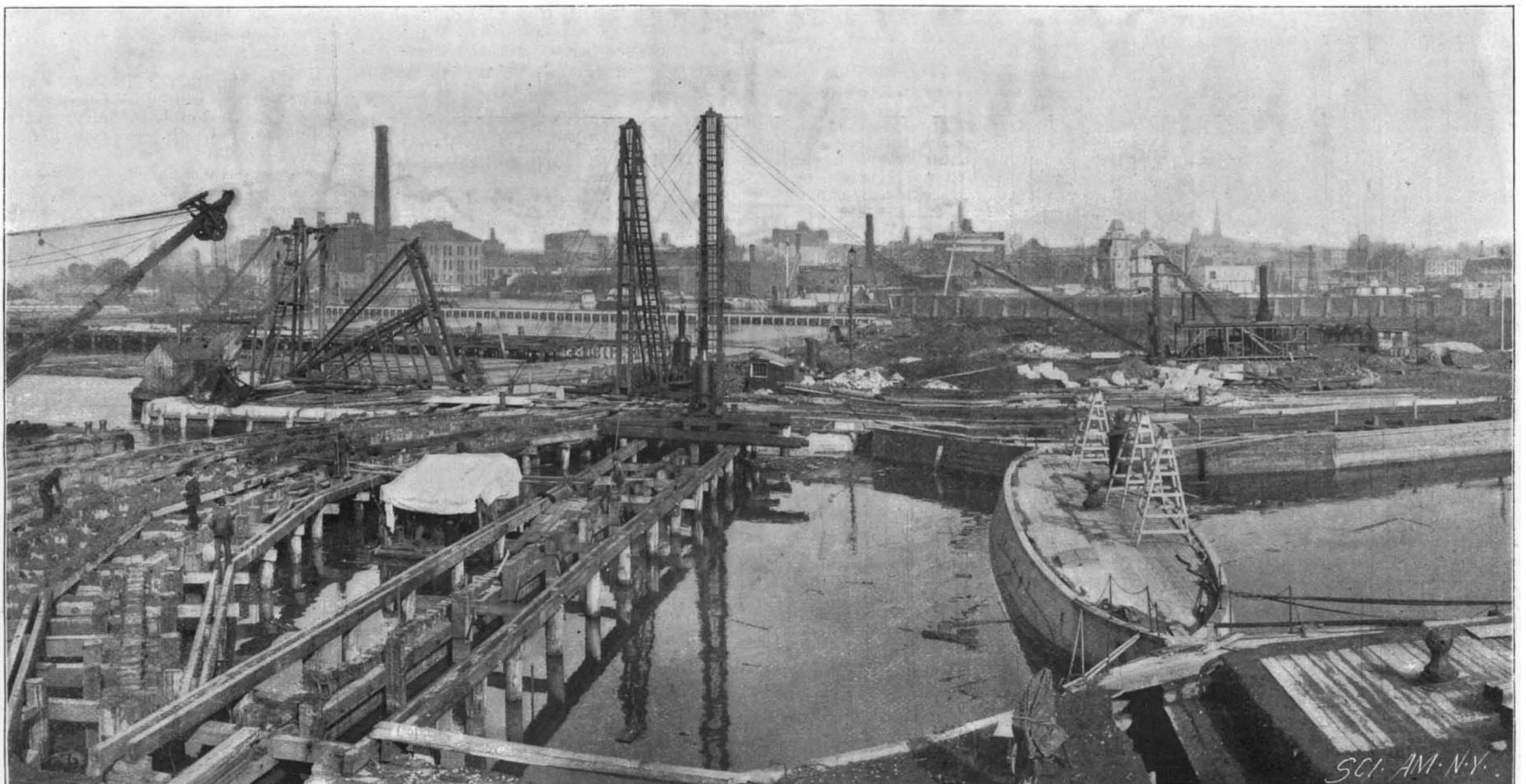
4.—COFFERDAM ACROSS ENTRANCE CHANNEL—DRY DOCK No. 3, BROOKLYN NAVY YARD.
