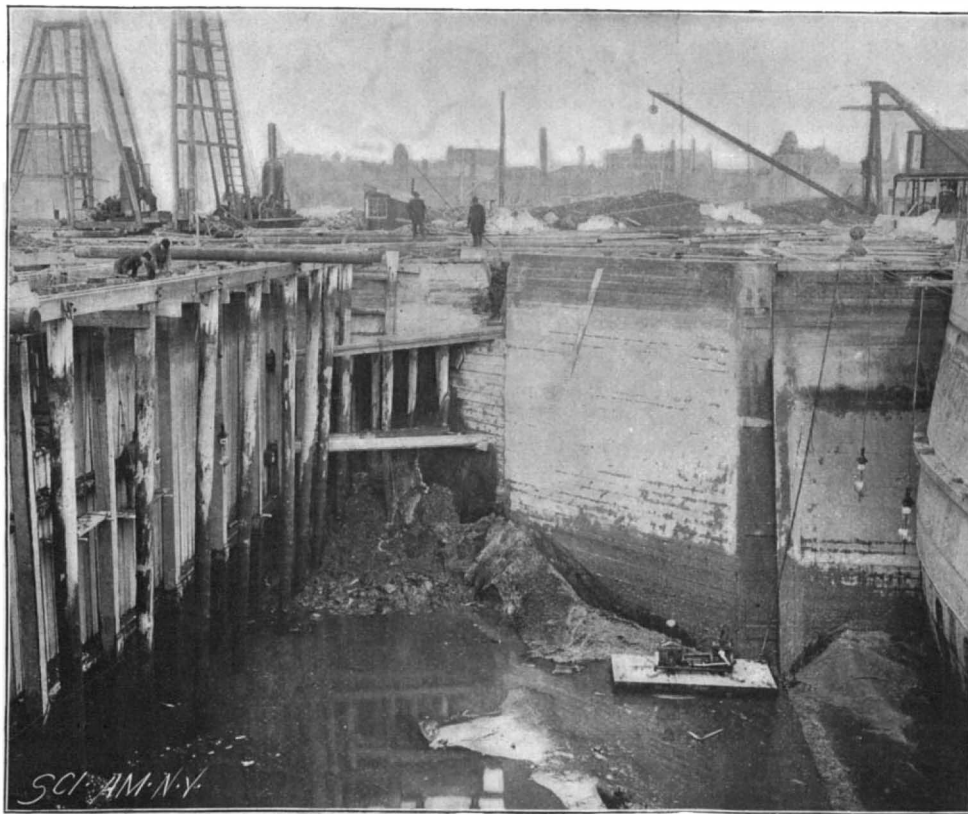
2.—BOTTOM OF DOCK ENTRANCE BETWEEN COFFERDAM AND CAISSON, SHOWING LOCATION OF LEAK.
