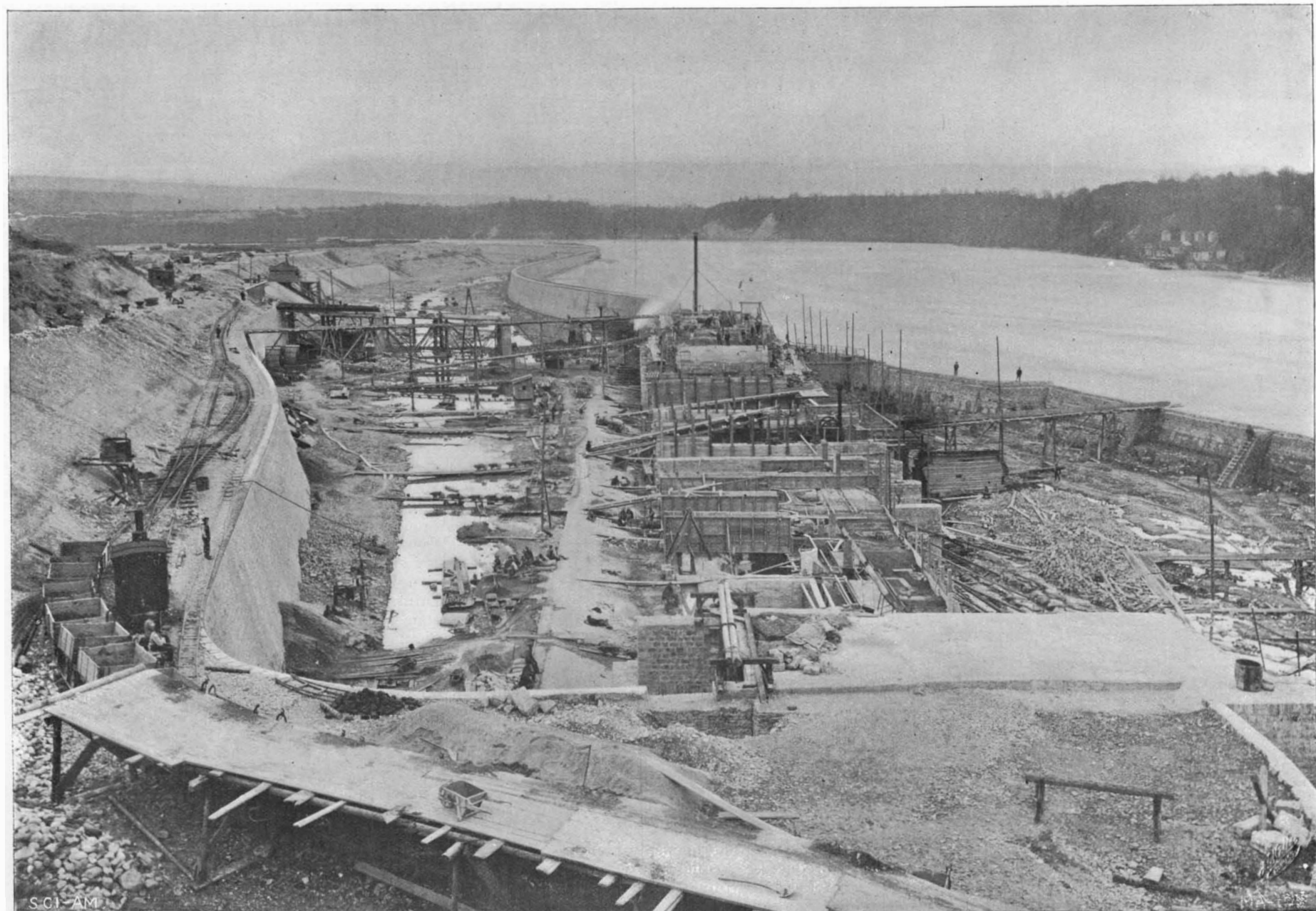
THE CONSTRUCTION OF THE POWER HOUSE OF THE RHEINFELDEN ELECTRICAL POWER PLANT—VIEW LOOKING UP THE HEAD RACE.
