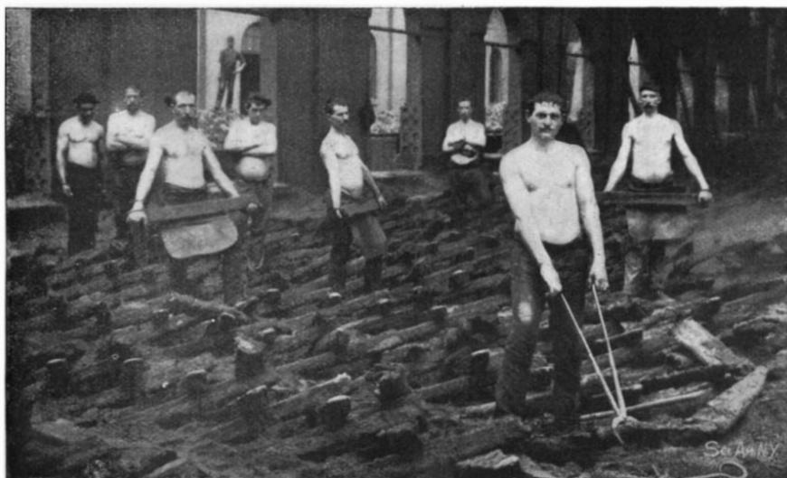
REMOVING PIG IRON FROM THE SAND.
