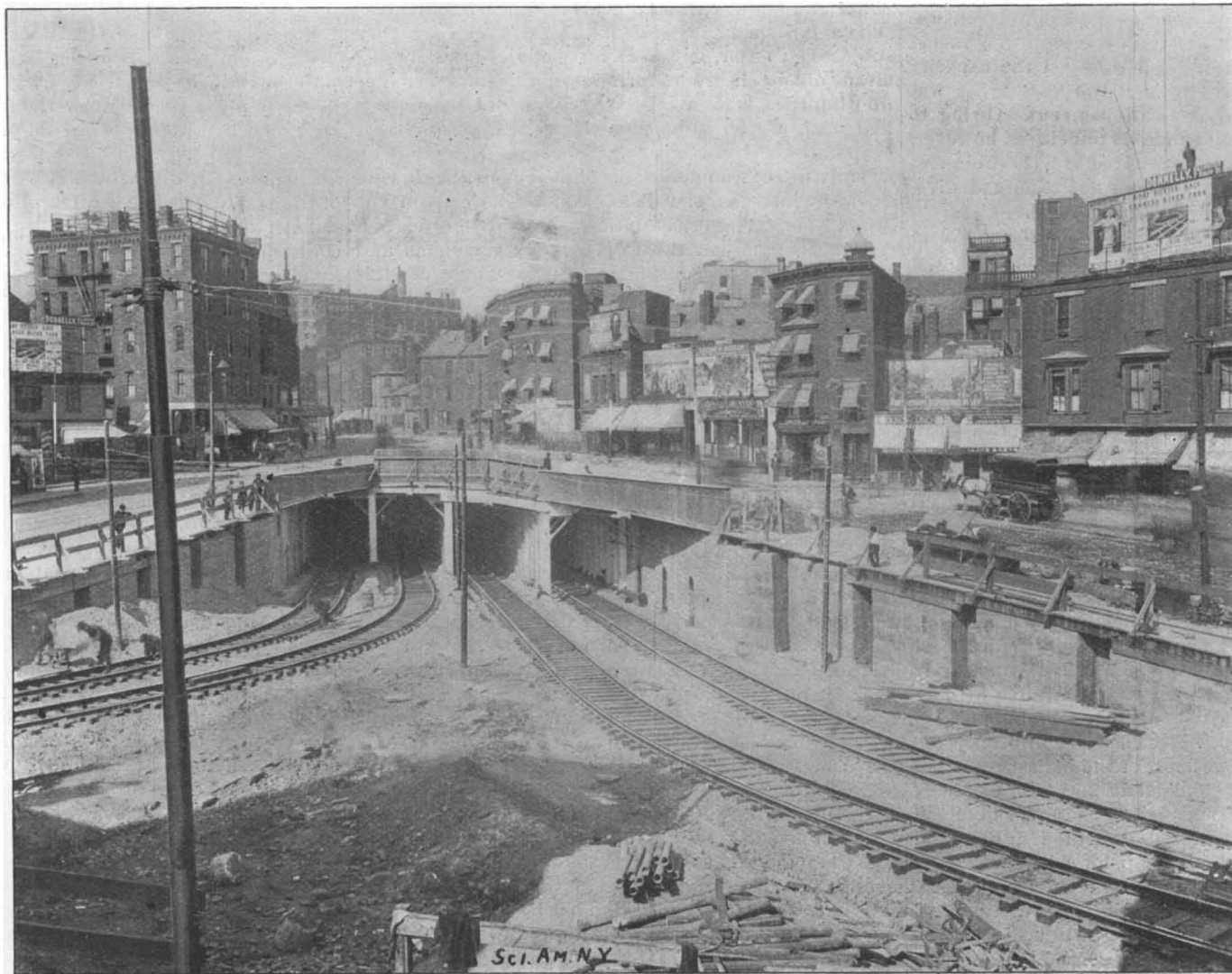
THE OPEN CUT, SHOWING TRACKS FOR TREMONT AND SHAWMUT AVENUE CARS,
