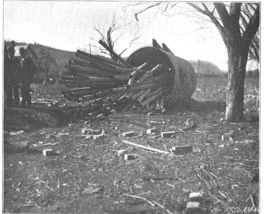
ONE-HALF OF BOILER IN FIELD 180 FEET DISTANT.
